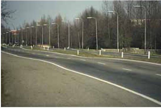
Figure 10: Longitudinal deformations due to settlements.
