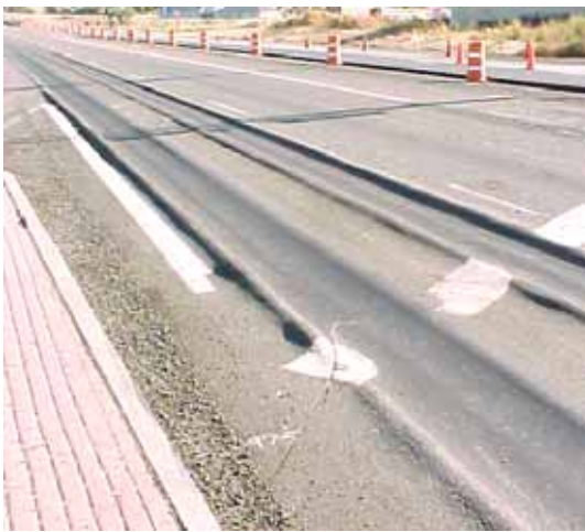
Figure 11: Rutting in an asphalt pavement.
