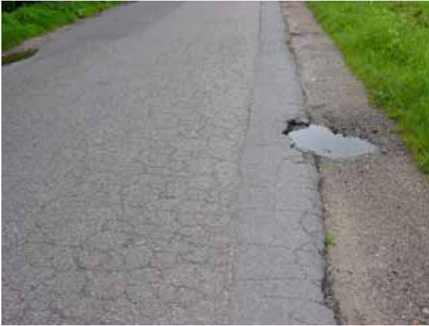
Figure 3: Cracking observed on a narrow polder road in the Netherlands.
