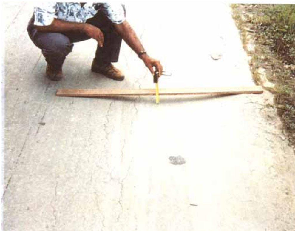
Figure 98: Excessive pavement deformation due to deformation of the unbound base and/or sub-base layer.
