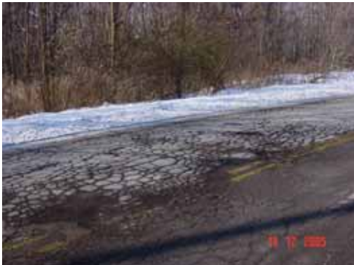
Figure 8: Roughness due to severe cracking.
