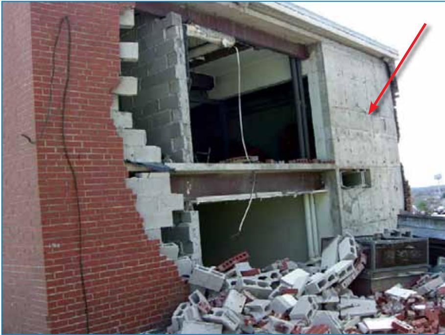
**Figure 4-148:** Collapsed brick veneer/CMU wall at a mechanical room. The cast-in-place concrete wall (arrow) remained, but the brick veneer was blown away.
