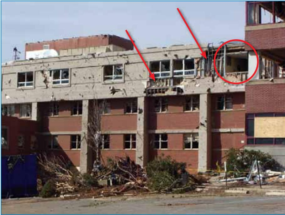
**Figure 4-145:** One window frame was blown away (red circle). The EIFS was penetrated by many missiles, and in some areas, the entire wall (except the studs) was blown away (arrows).
