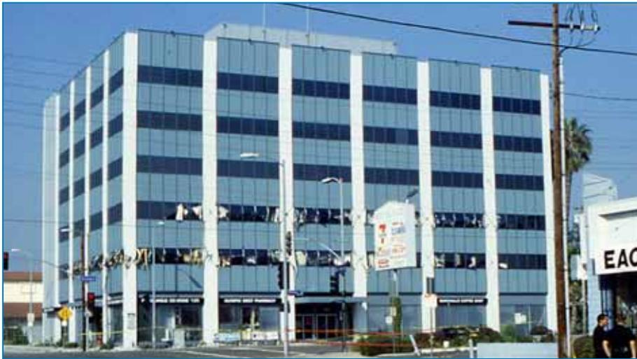
**Figure 2-16:** This concrete building suffered severe damage to the columns at the second floor level. It was deemed unsafe by the local jurisdiction and later demolished.
