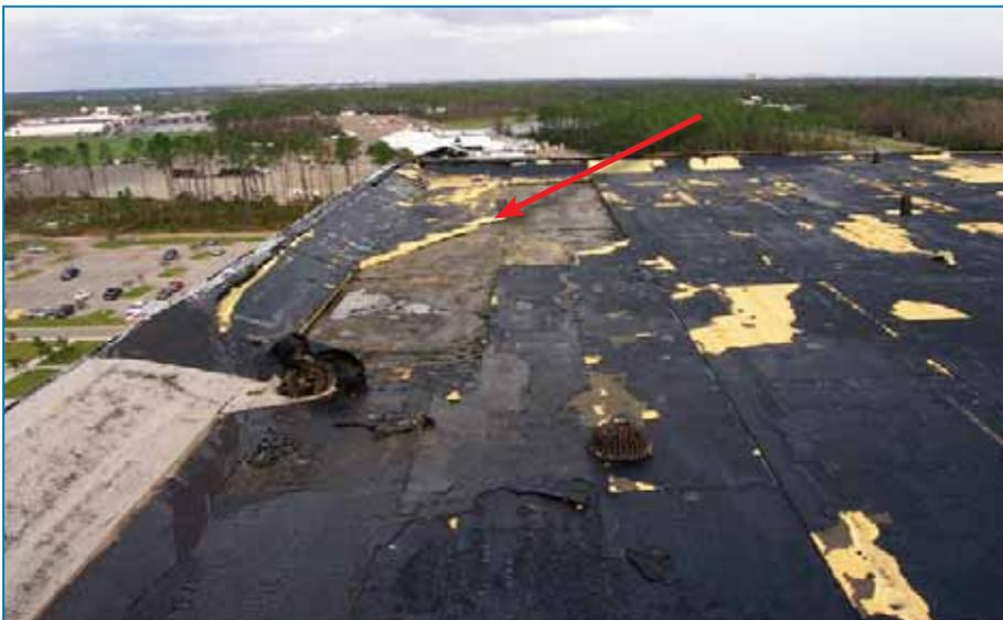
**Figure 4-71:** The blown off insulation (red arrow) may have initiated blow off of the roof membrane. Hurricane Ivan (Florida, 2004)
