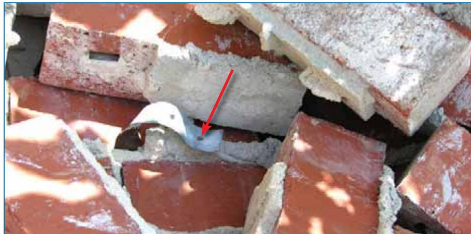
Ties are often installed before brick laying begins. When this is done, ties are often improperly placed above or below the mortar joints. When misaligned, the ties must be angled up or down to be embedded into the mortar joints (Figure 4-54). Misalignment not only reduces the embedment depth, but also reduces the effectiveness of the ties, because wind forces do not act in parallel direction to the ties.
