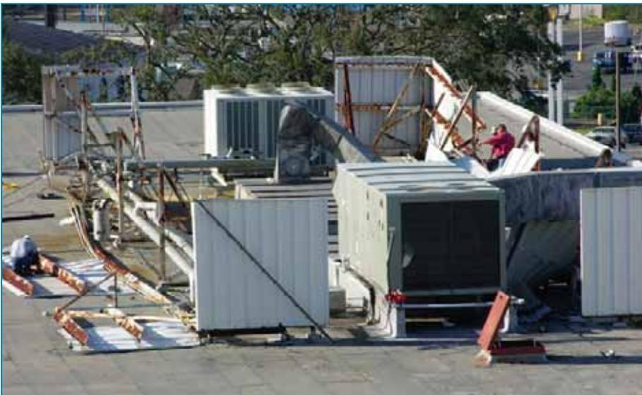
**Figure 4-94:** Equipment screen panels, such as these blown away at a hospital, can break glazing, puncture roof membranes, and cause injury. Hurricane Ivan (Florida, 2004)
