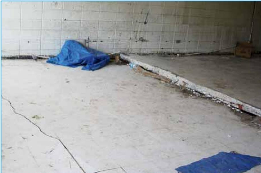
**Figure 3-15:** Concrete slab ruptured by hydrostatic pressure (buoyancy) induced by the floodwaters of Hurricane Katrina (2005).
