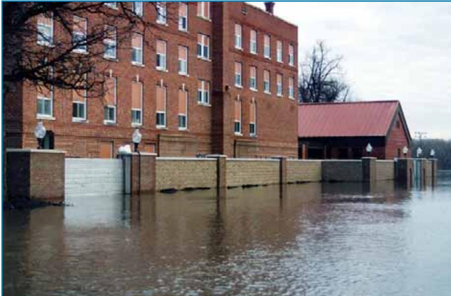
**Figure 3-39:** A masonry floodwall with multiple engineered openings in Fargo, ND during flooding in 2001.
