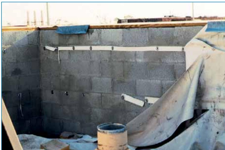
**Figure 4-70:** If mechanically attached base flashings have an insufficient number of fasteners, the base flashing can be blown away. Hurricane Andrew (Florida, 1992)
