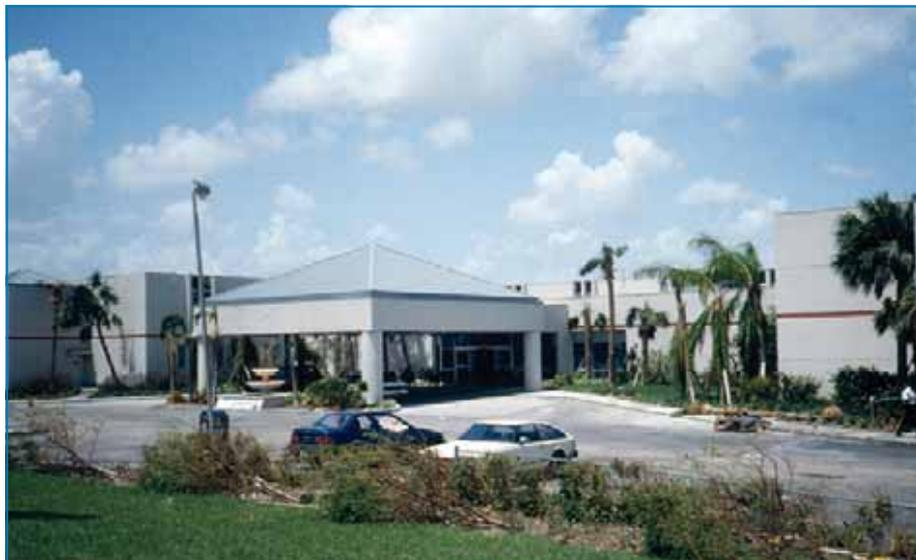
The 200-bed Deering Hospital opened shortly before Hurricane Andrew struck south Florida in 1992. Aggregate from the hospital's built-up roofs broke several windows, the roof covering was blown off in some areas (Figure 4-9), and the entrance doors at the emergency room were blown away. Because of extensive interior water damage, the entire hospital was evacuated after the storm and remained closed for 9 months.
