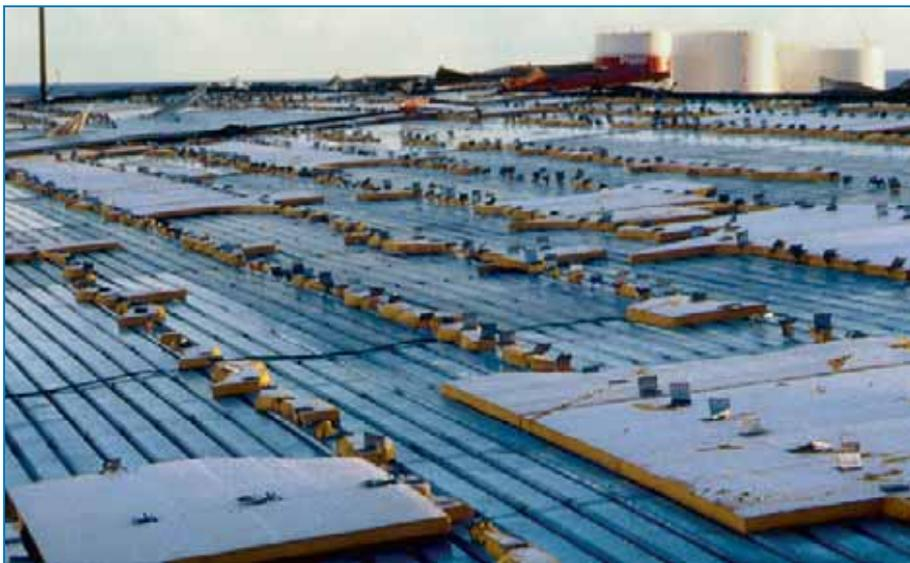
**Figure 4-73:** Significant interior water damage and facility interruption occurred after the standing seam roof blew off. Hurricane Marilyn (U.S. Virgin Islands, 1995)
