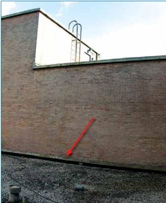
**Figure 4-58:** Water leaked inside along the base of the brick veneer walls (red arrow). Hurricane Katrina (Louisiana, 2005)
