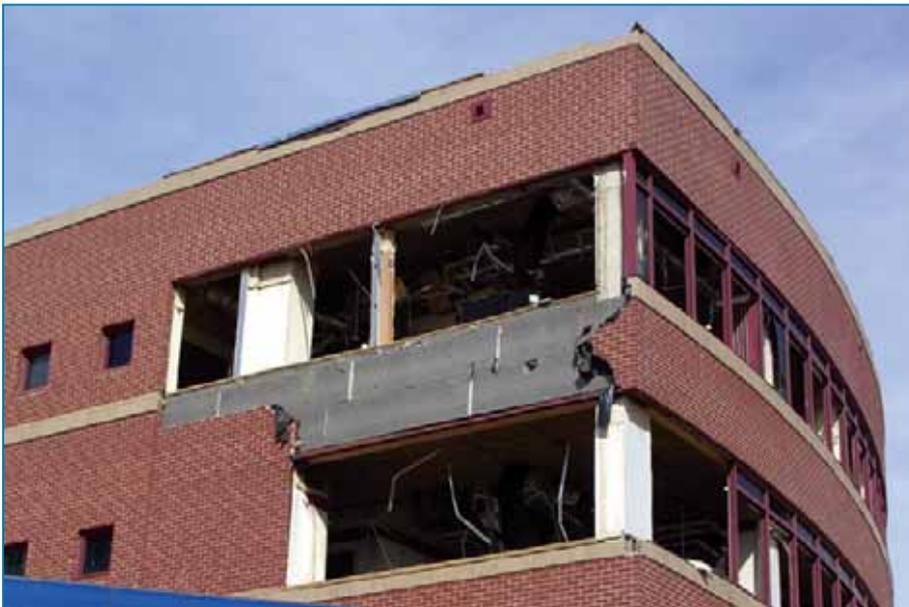
**Figure 4-146:** Several of the window frames were blown away, along with some of the brick veneer (1999 addition).
