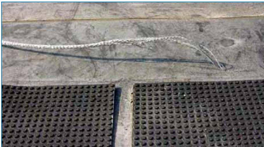
**Figure 4-99:** View of an end of a conductor at a hospital that became disconnected. Hurricane Katrina (Mississippi, 2005)
