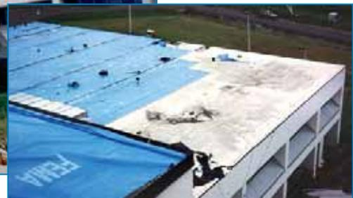
**Roof:** Roof covering damage (including rooftop mechanical, electrical, and communications equipment) is the most common type of wind damage, as illustrated by Figure 4-9. In addition to blowoff of the roof membrane (yellow arrow), ductwork blew away (red circle), a gooseneck was blown over (red arrow), and wall panels at an equipment enclosure were blown off (blue arrow). The cast-in-place concrete deck kept most of the water from entering the hospital.
