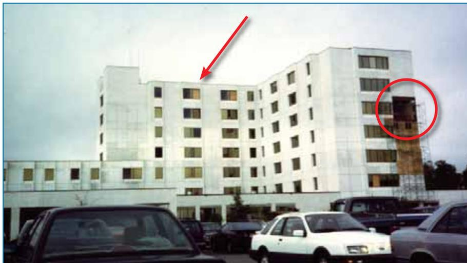
**Figure 4-11:** Collapse of non-load-bearing wall (red circle) and broken glazing from roof aggregate (red arrow). Hurricane Hugo (South Carolina, 1989)
