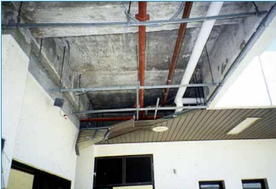
**Figure 4-49:** This suspended metal soffit was not designed for upward-acting wind pressure. Typhoon Paka (Guam, 1997)
