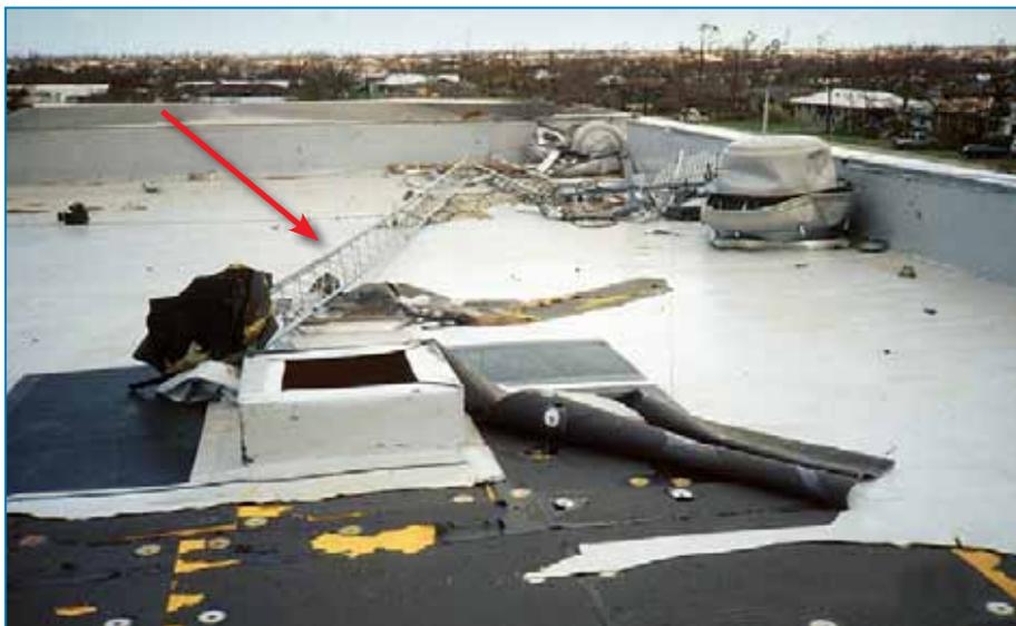
**Figure 4-95:** The collapse of the antenna tower caused progressive peeling of the roof membrane. Also note that the exhaust fan blew off the curb, but the high parapet kept it from blowing off the roof. Hurricane Andrew (Florida, 1992)
