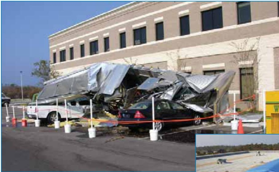
**Figure 4-86:** Although this 18,000-pound HVAC unit was attached to its curb with 16 straps, it blew off during Hurricane Ivan. (Florida, 2004)
