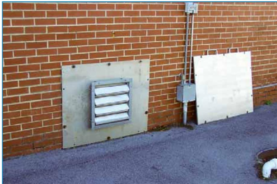
The frames that hold the floodproofing panels are permanently-mounted and sealed against the building to prevent seepage. The frames are designed with an aluminum cover to keep the channels free of dirt and debris. The metal panels that fit into the channels have rubber gaskets that are inspected each year as part of the hospital's routine maintenance program. The manufacturer recently advised replacement of the gaskets, as the 10-year anniversary of installation nears.
