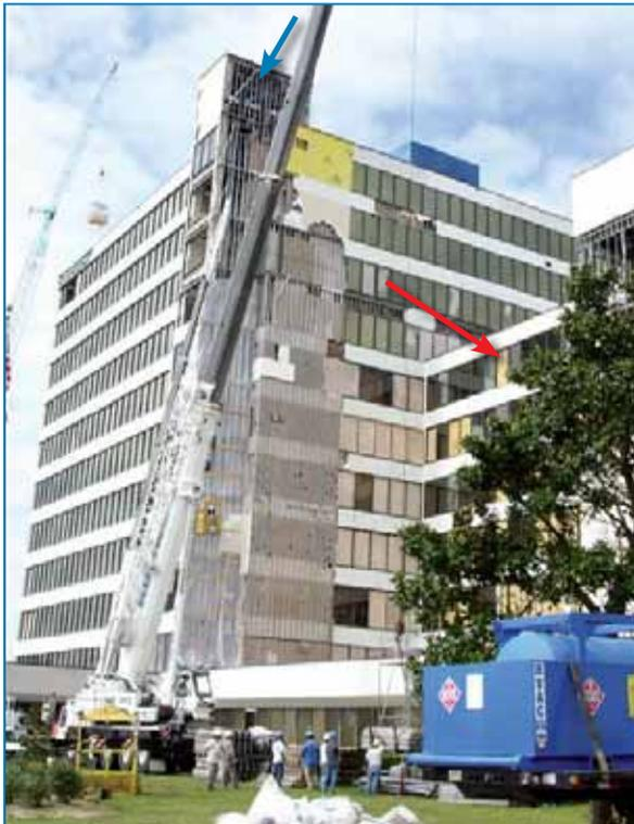
**Figure 4-18:** Broken windows in the connecting walkway between the hospital (right) and MOB (left) (red arrow). Also note the broken windows and loss of EIFS (including the gypsum board on both sides of the studs) at the elevator enclosure (blue arrow).
