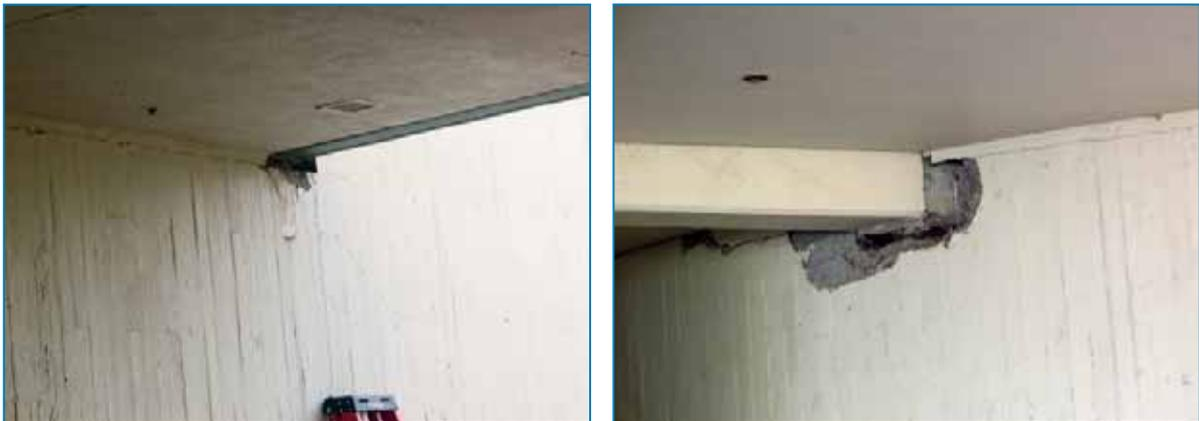
Figure 2-40: Spalling at beam connections
