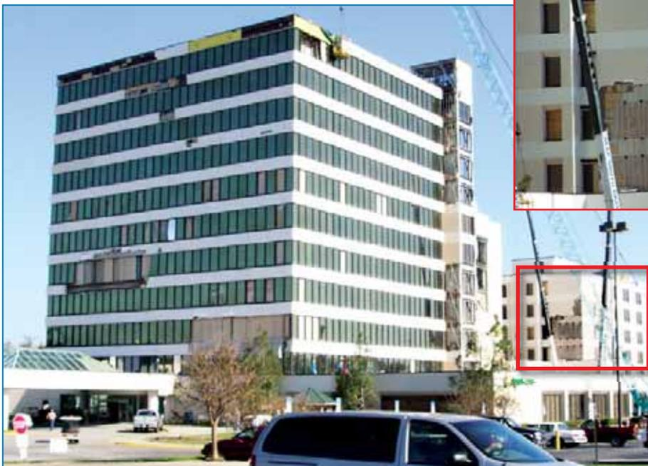
**Figure 4-19:** EIFS debris blown off the hospital building (Item J on Figure 4-13) in the background (red square) broke numerous windows in the MOB (item G on figure 4-13) in the foreground.
