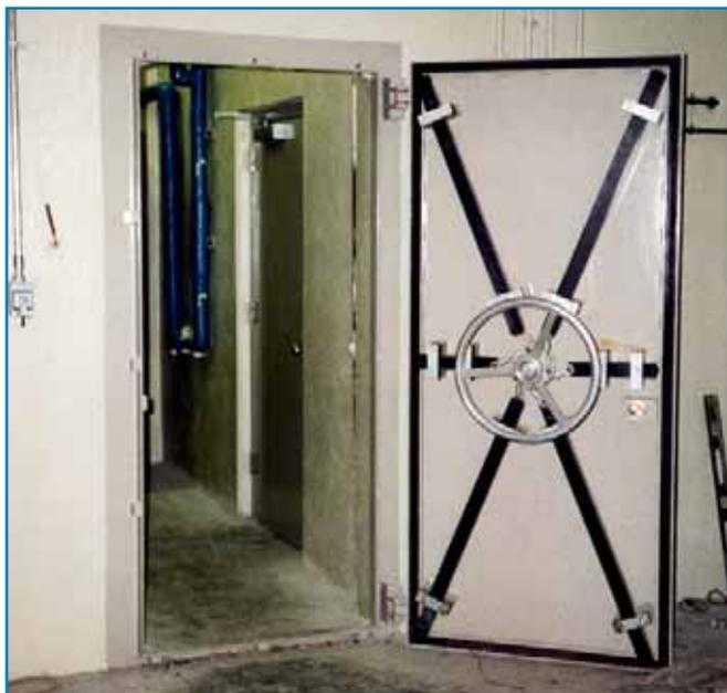
**Figure 3-36:** Permanent watertight doors designed for deep water
