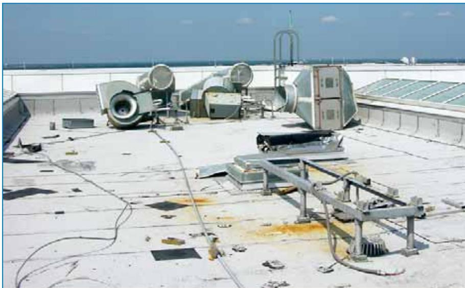
**Figure 4-25:** Temporary coverings placed over two large openings in the roof that were left after the ductwork blew away. Hurricane Katrina (Mississippi, 2005)
