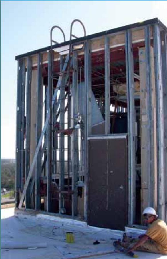
**Figure 4-22:** The only remaining portion of the exterior wall surrounding the elevator penthouse on the MOB was the steel studs.
