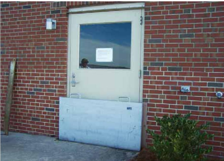
**Figure 3-46:** Most of the panels can be installed by hand. Note the protective metal strip leaning against the building on the left; normally this strip covers the horizontal channel into which the panel is inserted.
