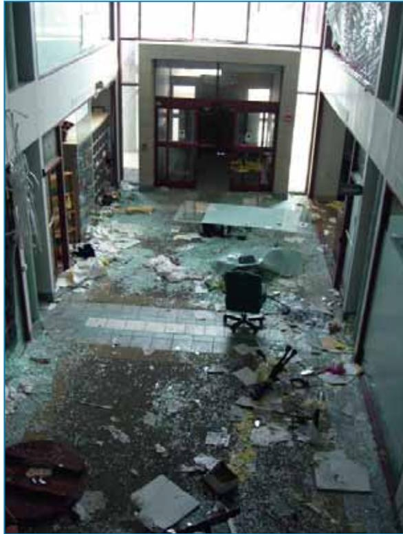
Damage also occurred on other facades, including collapse of a glass curtain wall and a portion of a brick veneer/unreinforced CMU wall (Figure 4-148). A large unreinforced brick chimney collapsed on a roof, and a large rooftop air handling unit (20 x 7 x 9 feet) was shifted several feet. A substantial amount of water entered the building at various places where the envelope was breached.
