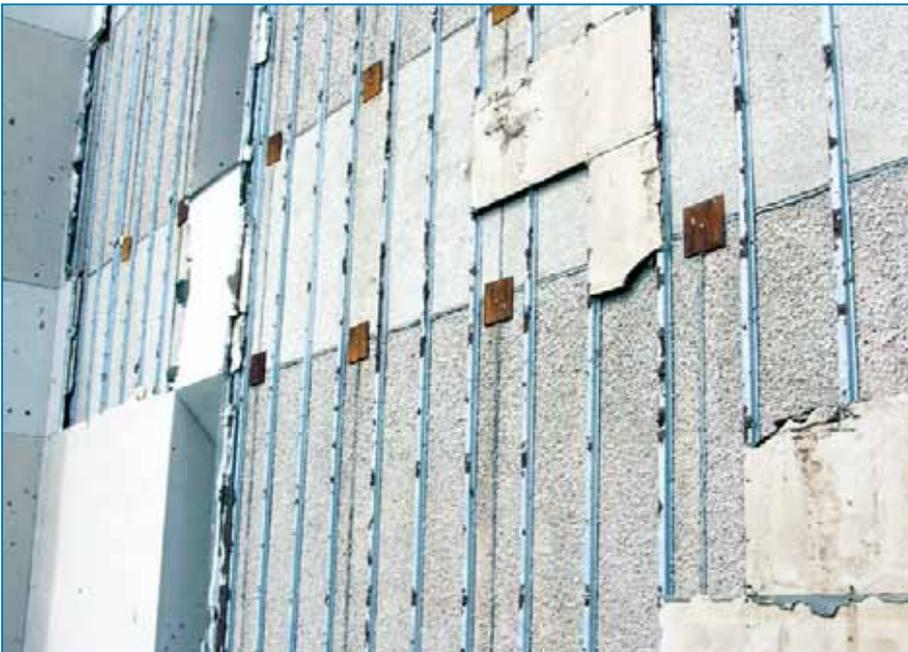
**Figure 4-23:** Close-up of the damaged EIFS at the hospital. In this area most of the insulation and gypsum board was blown from the steel furring channels.
