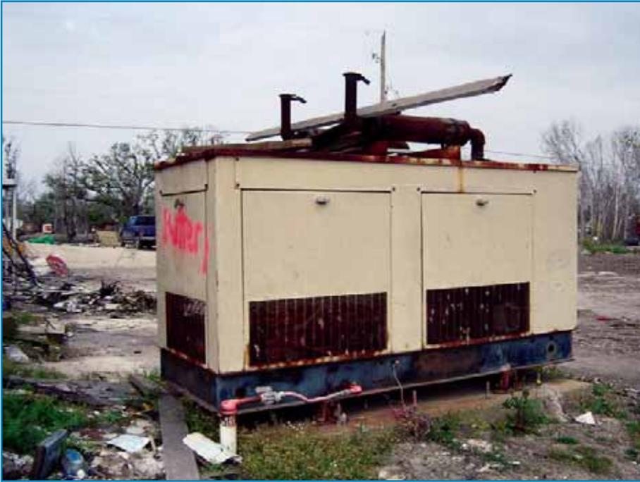
**Figure 3-21:** Although it was anchored and not displaced by floodwaters, this generator was out of service after being submerged (Hurricane Katrina, 2005).
