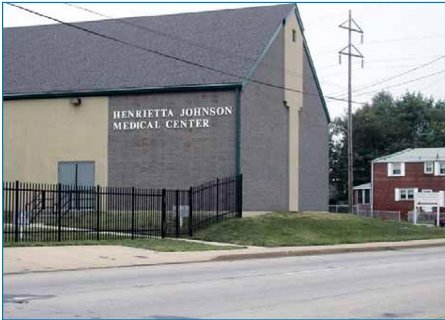
**Figure 3-27:** Structural fill was placed to elevate the Henrietta Johnson Medical Center above the shallow flood hazard area in Wilmington, DE.
