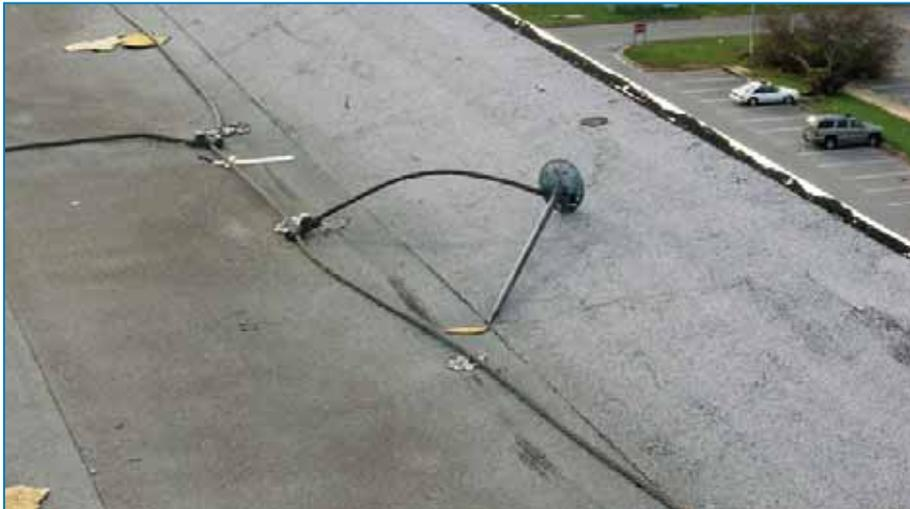
**Figure 4-98:** An air terminal debonded from the hospital’s roof. Displaced air terminals can puncture tough membranes, such as this modified bitumen membrane. Hurricane Ivan (Florida, 2004)
