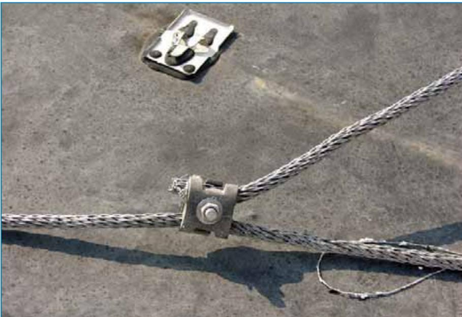
**Figure 4-105:** Bolted splice connectors are recommended to prevent free ends of connectors from being whipped around by wind. Hurricane Katrina (Mississippi, 2005)
