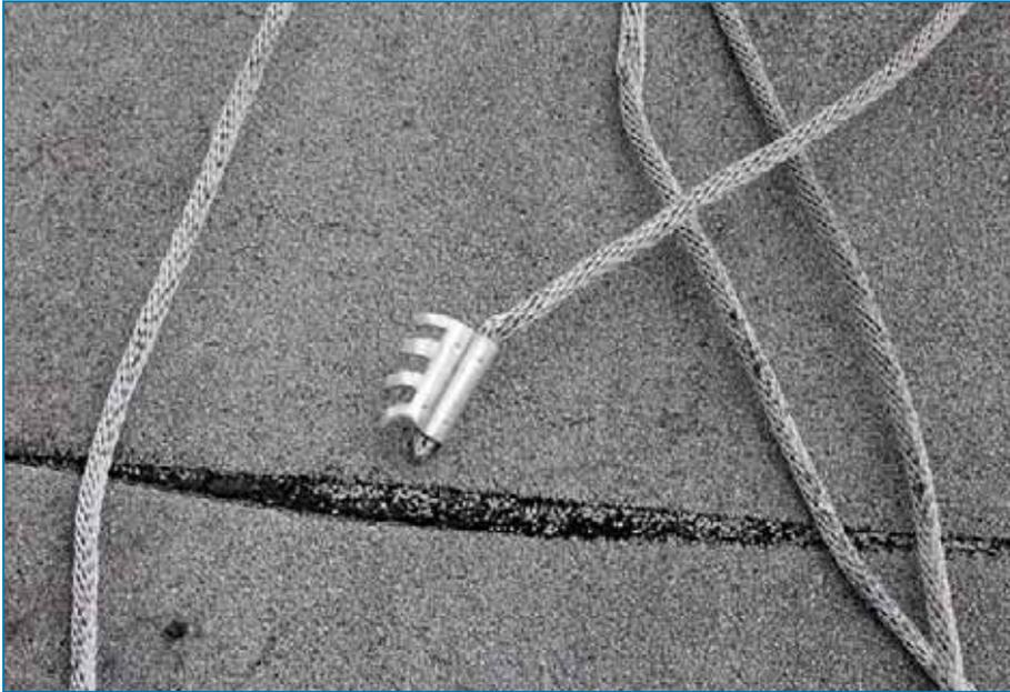
**Figure 4-104:** If conductors detach from the roof, they are likely to pull out from pronged splice connectors. Hurricane Charley (Florida, 2004)
