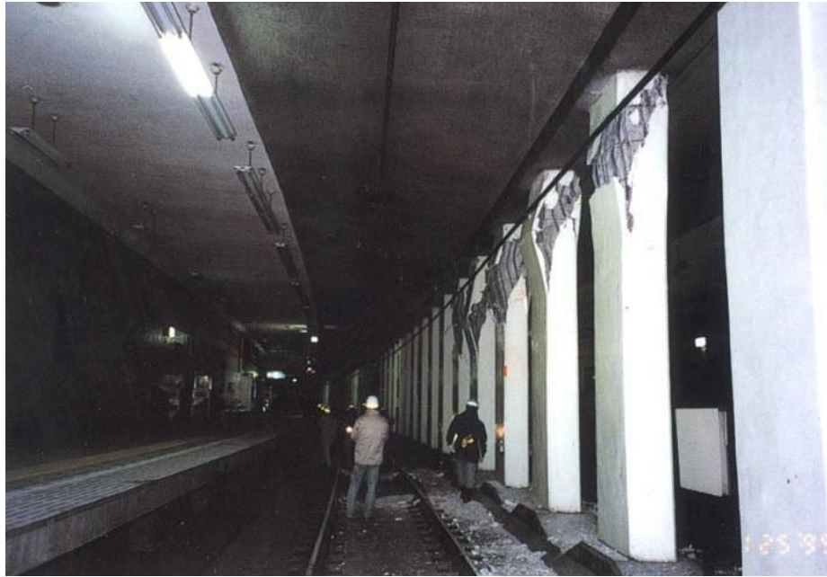
Figure 13-11 Shear Failure at Top of Columns of Cut-and-Cover Tunnel Between Daikai and Nagata Stations - 1995 Kobe Earthquake, Japan
