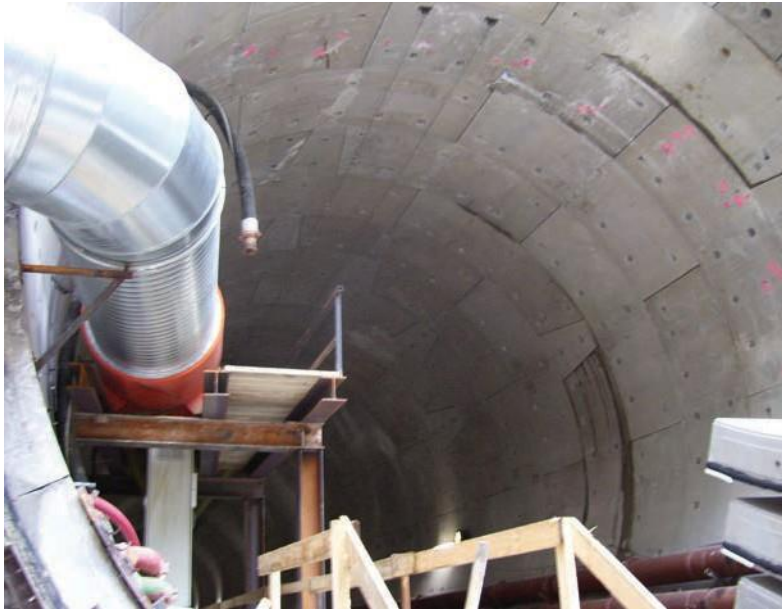
Figure 10-2 Precast Segmental Lining
