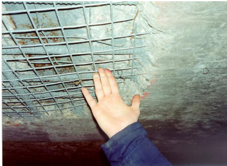
Figure 16-12 Reinforcing Steel for Repair, Sumner Tunnel Boston
