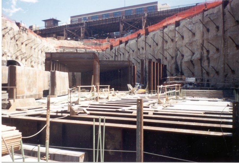
Figure 5-6 Tie-back Excavation Support leaves Clear Access
