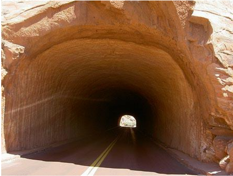
Figure 6-36 Unlined Rock Tunnel in Zion National Park, Utah
