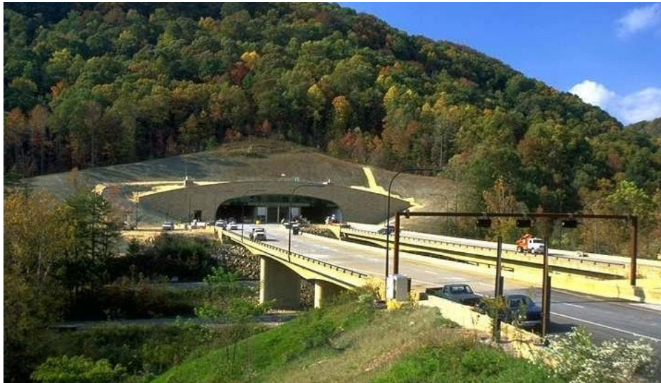
Figure 2-8 Portal Structure for Cumberland Gap Tunnel
