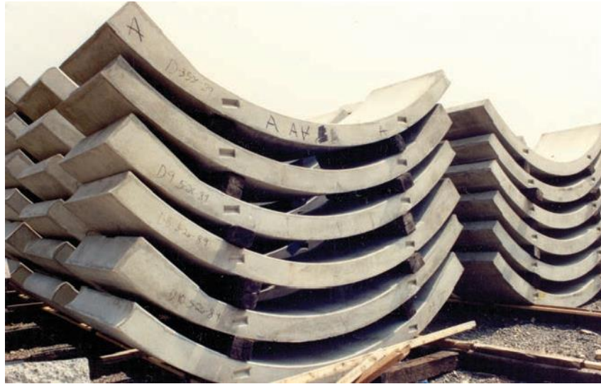
Figure 10-9 Stacked Precast Segments for Two-Pass Lining
