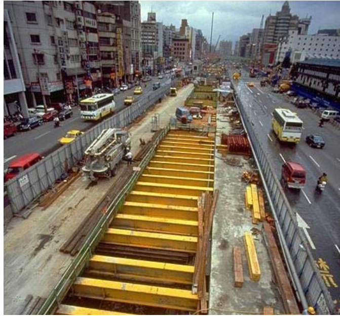
Figure 5-7 Braced Slurry Walls
