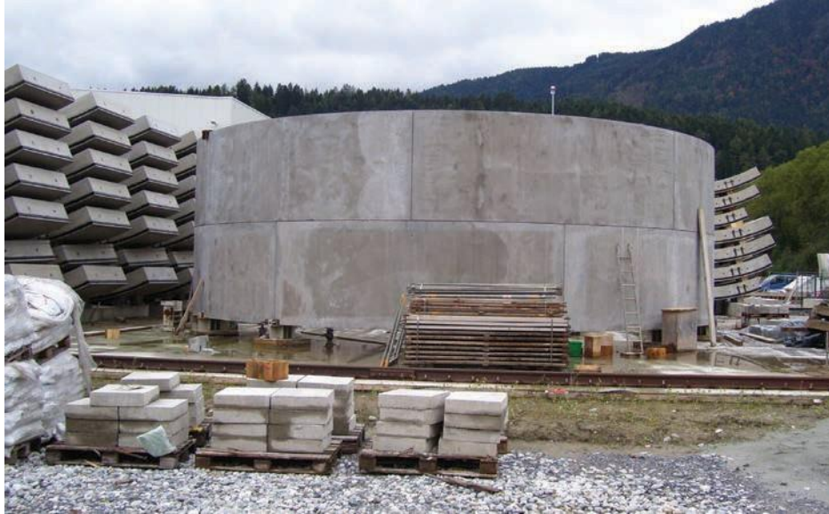
Figure 10-13 Mock-up of Precast Segment Rings
