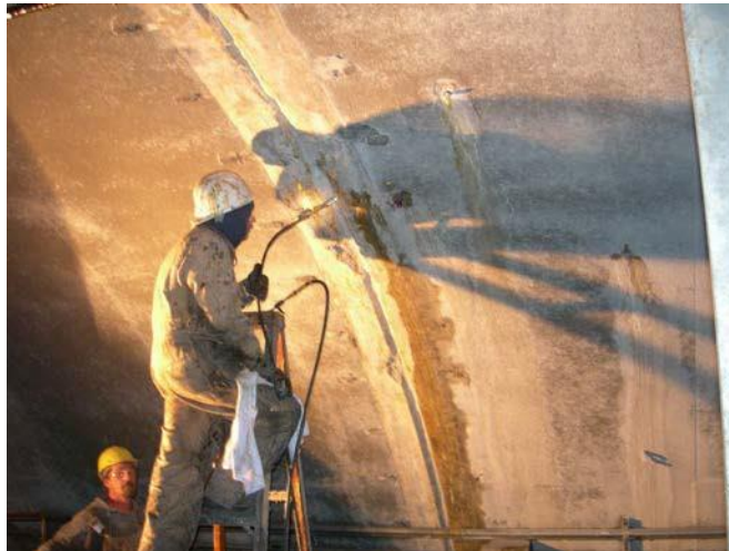
Figure 16-4 Leak Injection, Tuscarora Tunnel PA Turnpike
