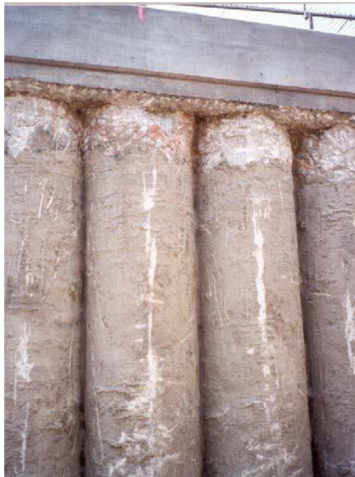
Figure 5-8 Tangent Pile Wall Construction Schematic
