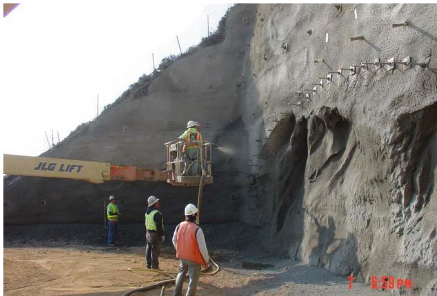
Figure 9-18 Pre-Support at Portal Wall and Application of Shotcrete for Portal Face Protection (Devil's Slide Tunnels, California)
