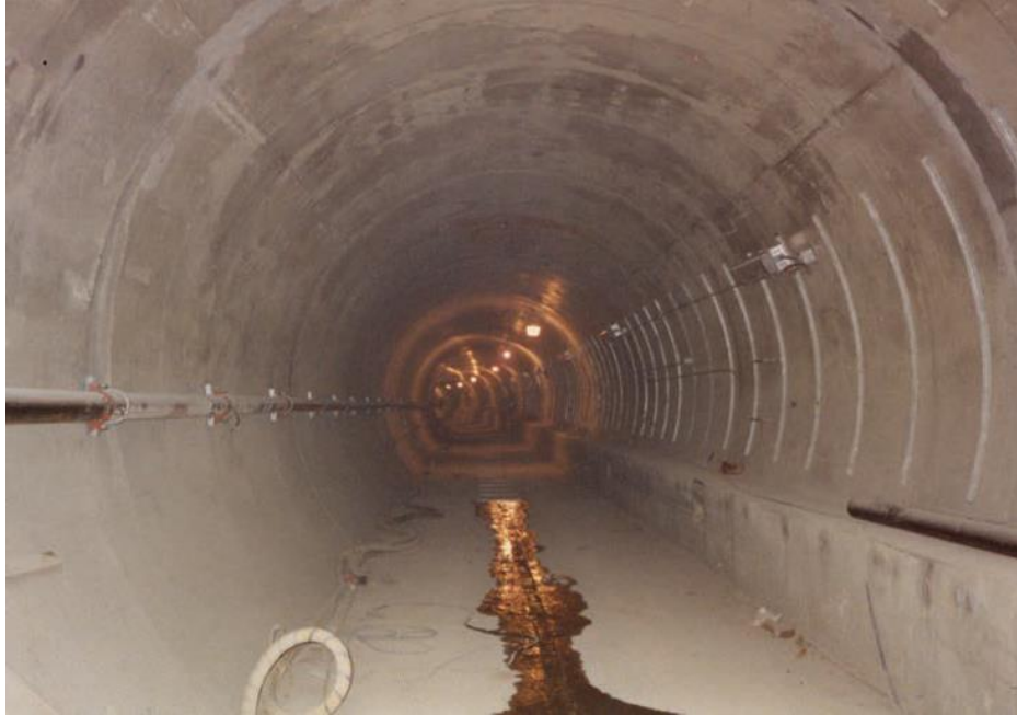
Figure 10-6 Cast-In-Place Concrete Lining, Washington DC
