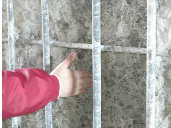
Figure 16-7 Substrate after Hydro-demolition, Shawmut Jct. Boston
