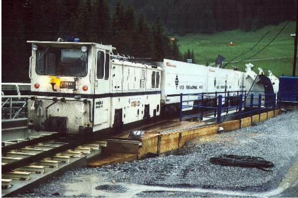
Figure 14-4 Muck Train Dumping at Portal
