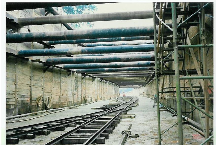
Figure 5-5 Braced Soldier Pile and Lagging Wall
