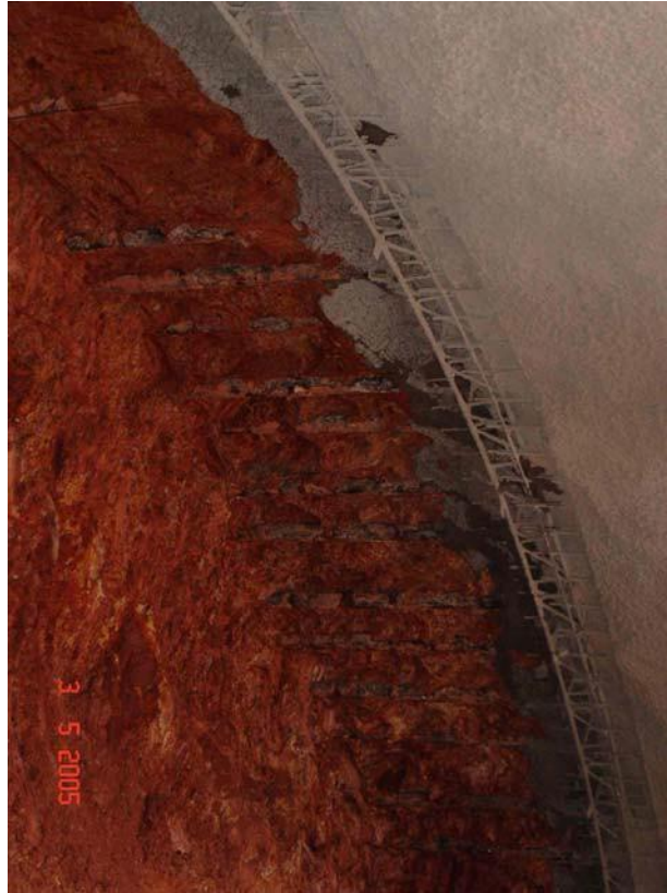
Figure 9-17 Pre-support by Pipe Arch Canopy, Exposed Steel Pipes Upon Excavation of a New Round (Fort Caning Tunnel, Singapore)
