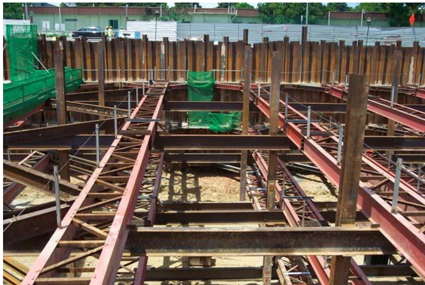
Figure 5-4 Sheet Pile Walls with Multi Level-Bracing
