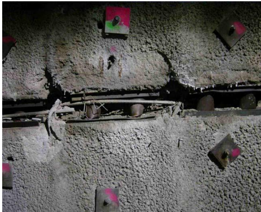
Figure 8-4 Yielding Support Crushed to 20 cm (One-half) (ILF, 2008)
