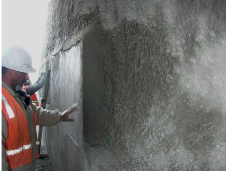
Figure 16-13 Shotcrete Finishing, Shawmut Jct. Boston
