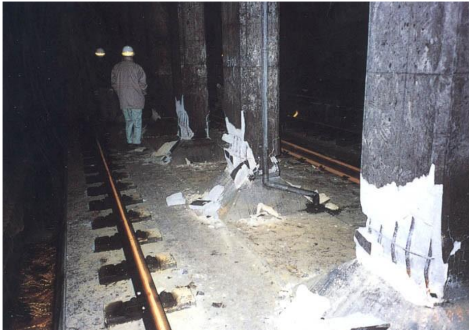
Figure 13-10 Fracture at Base of Columns of Cut-and-Cover Tunnel between Daikai and Nagata Stations - 1995 Kobe Earthquake, Japan
