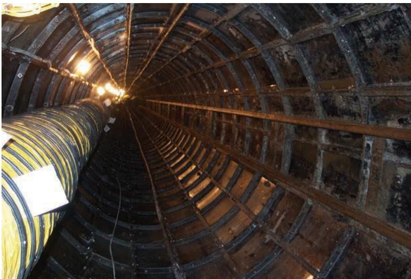
Figure 10-3 Baltimore Metro Steel Plate Lining
