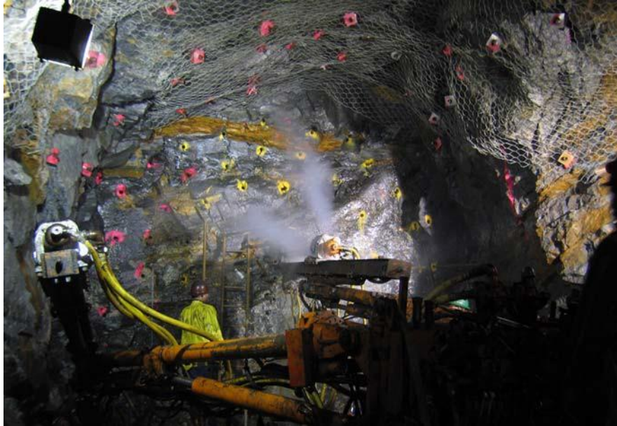
Figure 6-8 Drilling for a Tunnel Blast
