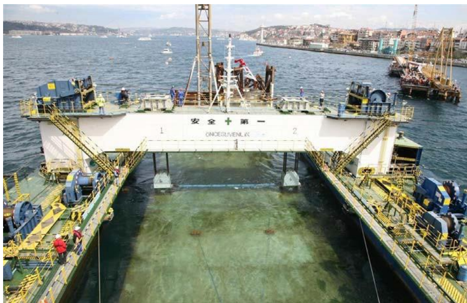
Figure 11-15 A Tunnel Element is Being Placed.
