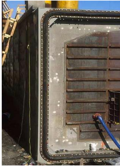
Figure 11-19 Gina-type Immersion Gasket at Fort Point Channel, Boston, MA
