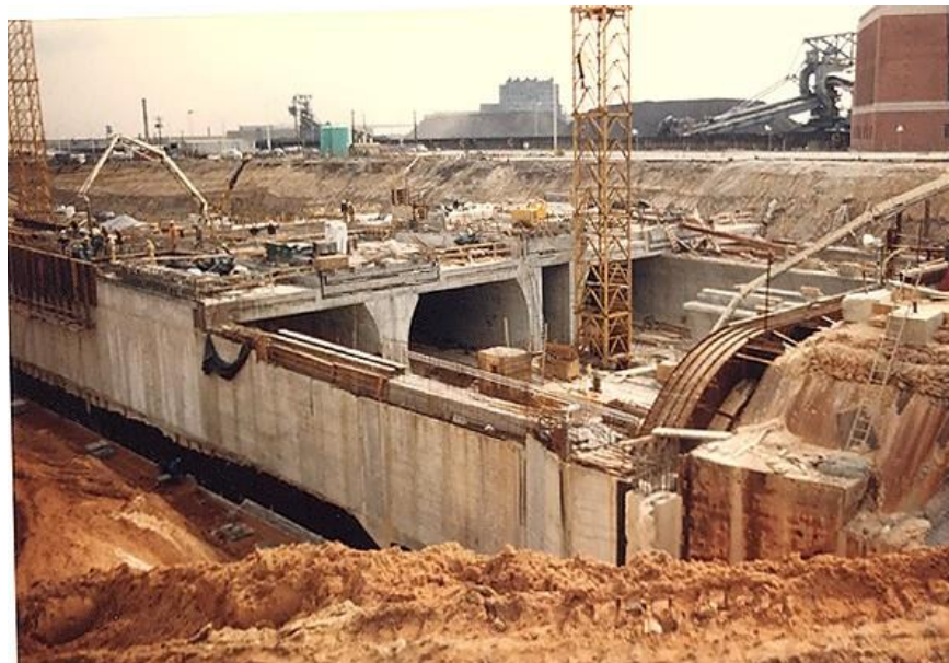
Figure 5-3 Cut and Cover Construction using Side Slopes Excavation- Ft McHenry Tunnel, Baltimore, MD
