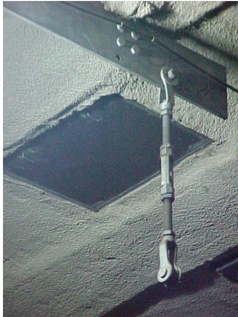
Figure 16-22 Typical Replacement Hanger Hardware
