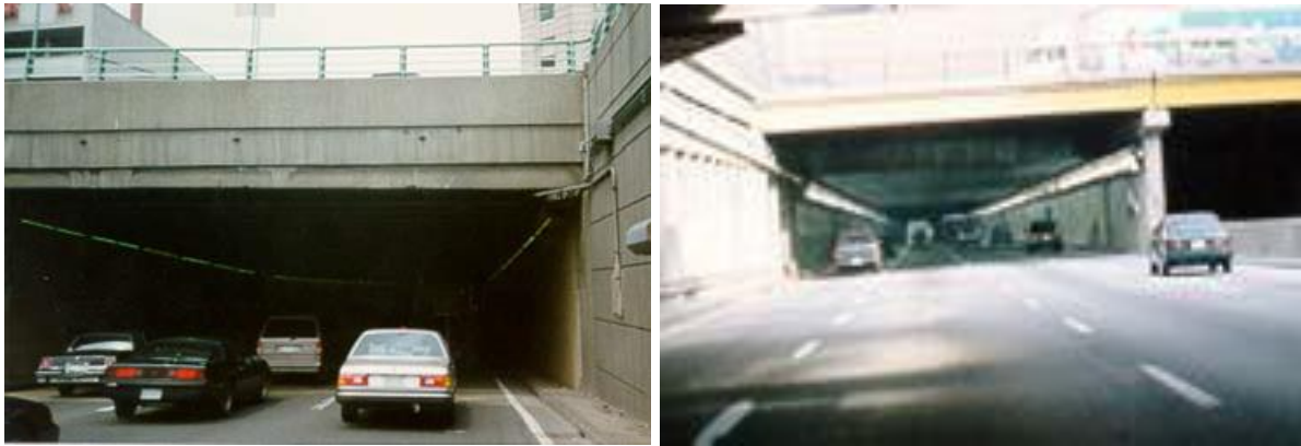
Figure 2-7 “Black Hole” (Left) and Proper Lighting (Right)
