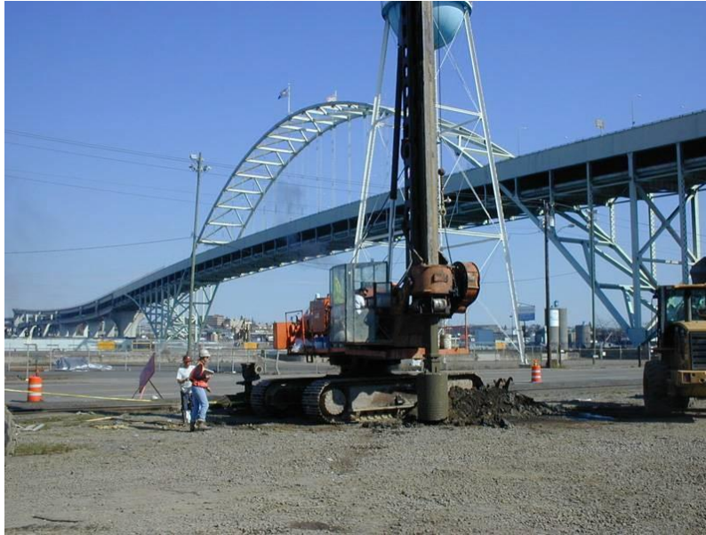
Figure 3-7 Rotasonic Sampling for a CSO Tunnel Project at Portland, Oregon.
