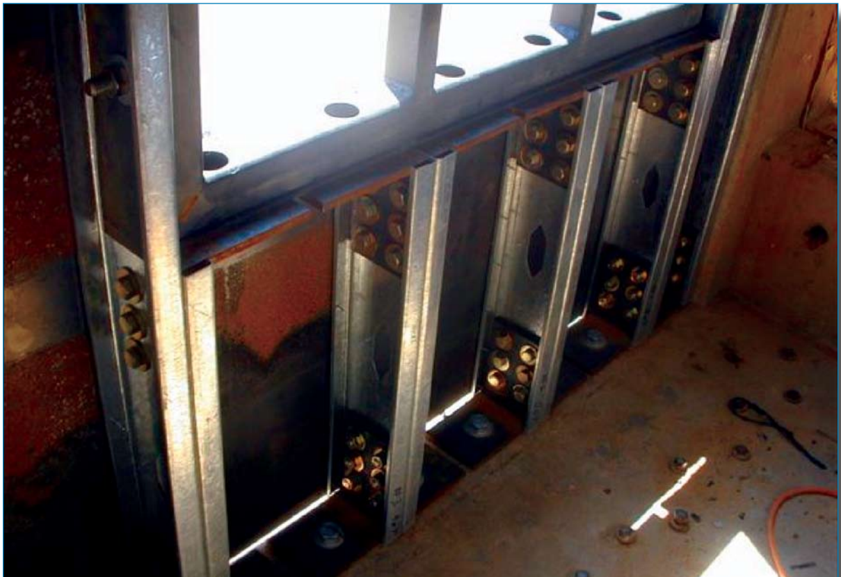
Figure 2-19 Metal stud blast wall
