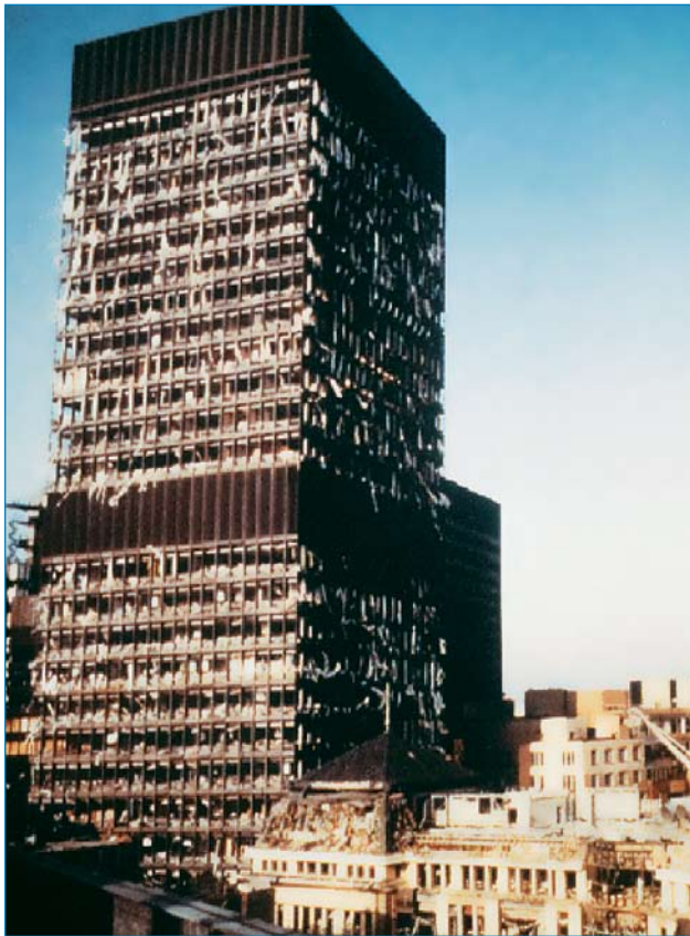
Figure 2-9 Blast damaged façade
