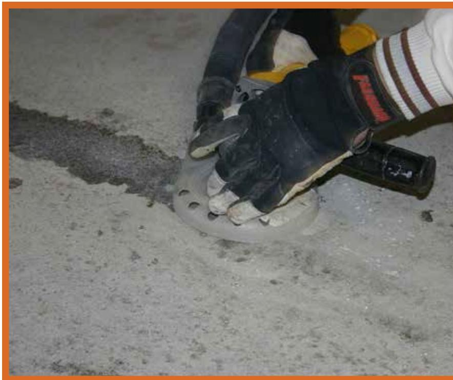
Thorough crack repair and efficient grinding are becoming commonplace prior to installing an overlay.
