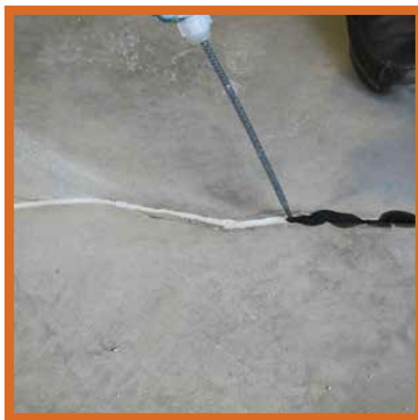
Epoxy crack fillers are popular for repairing cracks prior to overlay installation.
