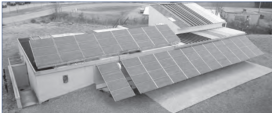
Figure 13. Building-integrated photovoltaic (BIPV)(offset-mounted) installed on the low-slope membrane roof systems and the south-facing wall of the ESRA.
