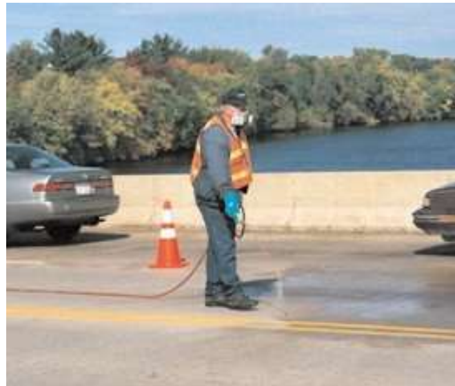
Fig12-12. Penetrating sealers help protect reinforcing steel in bridge decks from corrosion due to chloride infiltration without reducing surface friction. (69976)
