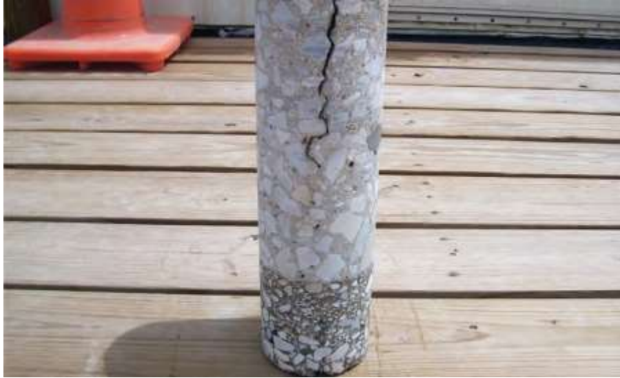
Figure 2. Deep Plastic Shrinkage Crack (below mid-depth)
