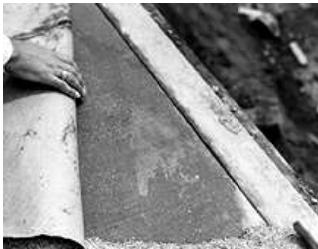
Fig.12-6. Impervious curing paper is an efficient means of curing horizontal surfaces. (69994)
