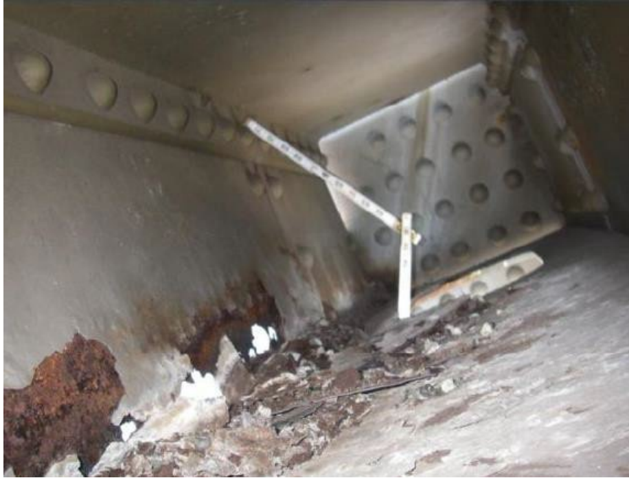
Figure 33. Photo. Inside of built-up box member.
