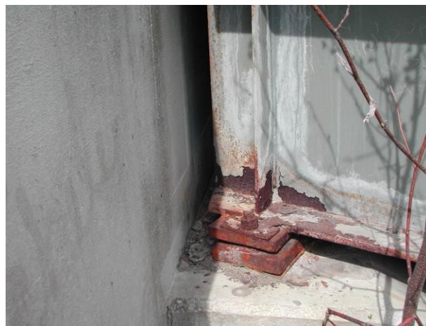
Figure 15. Photo. Deterioration of bearing area beneath a leaking joint with only single-coat inorganic zinc-rich paint.
