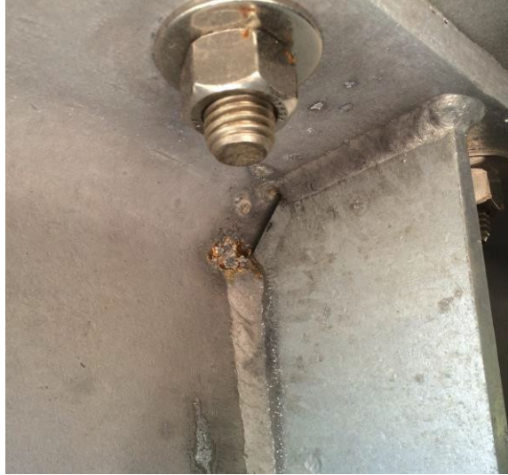
Figure 40. Photo. Connection plate welded to rolled I-beam along with corrosion emanating from unsealed weld.
