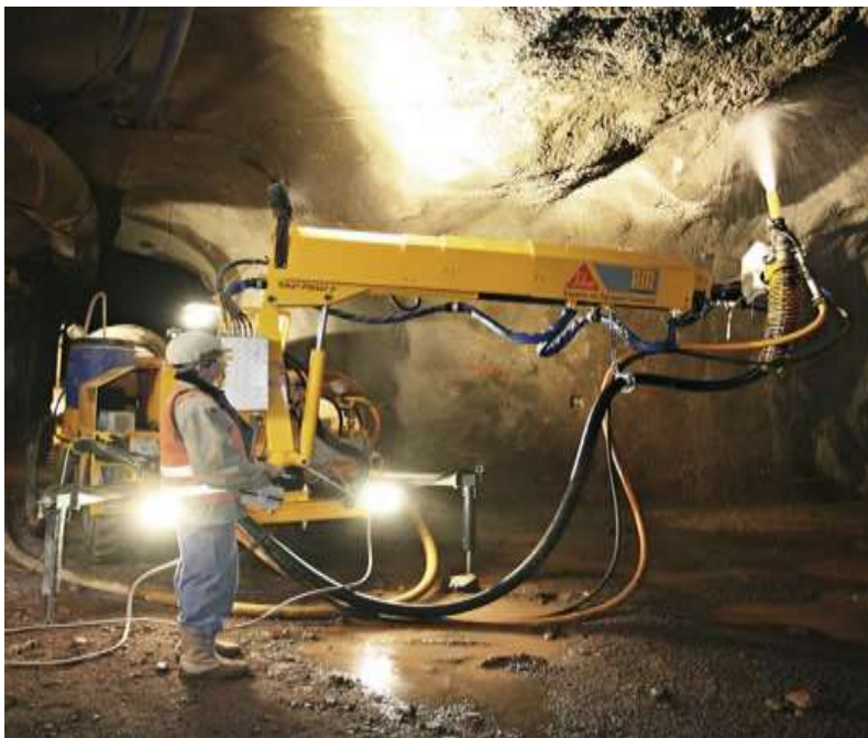
Figure 2.3. Shotcrete application in lining of the tunnel
