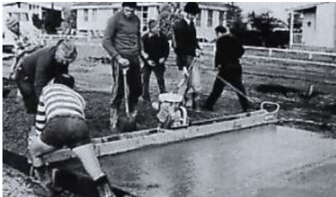
Figure 3.8. Typical surface vibrator.
