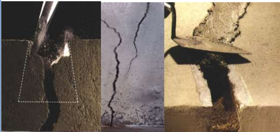
Figure 2.1. Repairing the cracks
