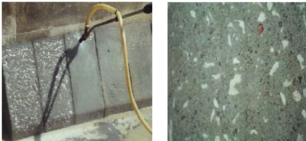
Figure 3.3. Substrate surface treated with sand blasting (Julio et al., 2004)
