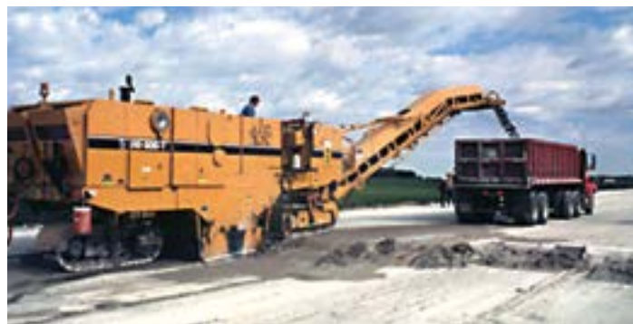
Figure 118. Typical concrete pavement milling operation (source: Randell Riley, Illinois chapter, ACPA)
