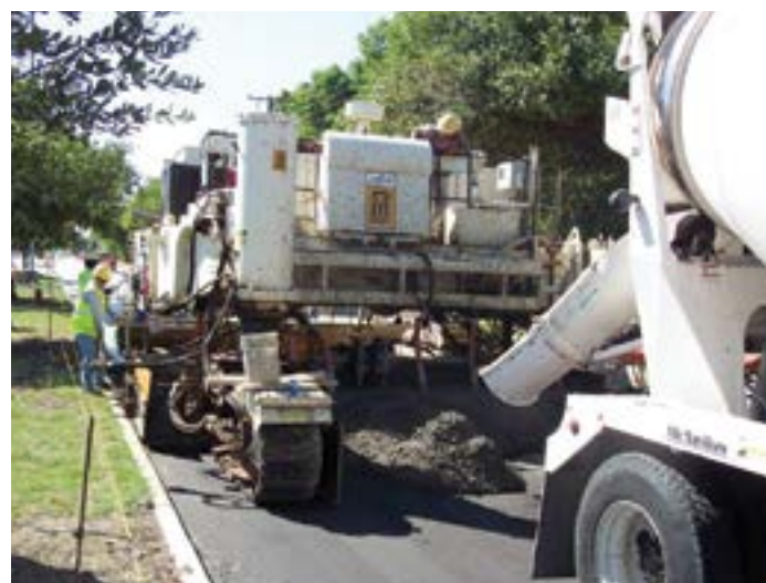
Figure 97. A typical four-track paver modified to three tracks, providing zero clearance in a C/G situation in Oklahoma (source: Jim Duit, Duit Construction Co., Inc.)
