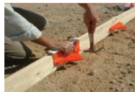
Figure 67. Taper-shaped construction joint plate dowel using fixed forms (source: Nigel Parks, PNA Construction Technology)
