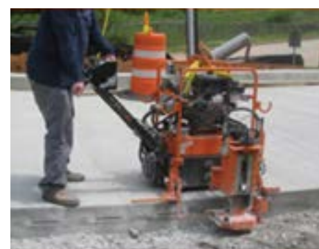
Figure 69. Slots being cut to accept the football-shaped plate dowels (source: Nigel Parks, PNA Construction Technology)
