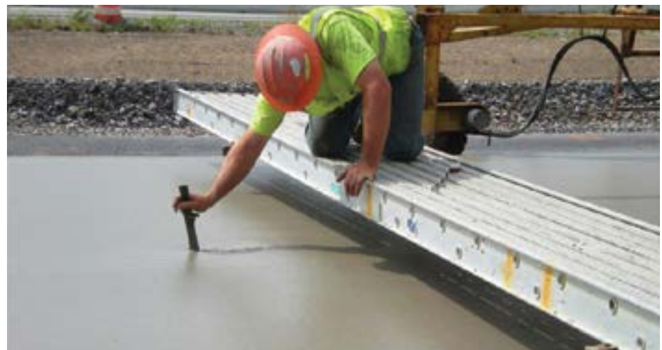
Figure 115. Manually verifying dowel placement
