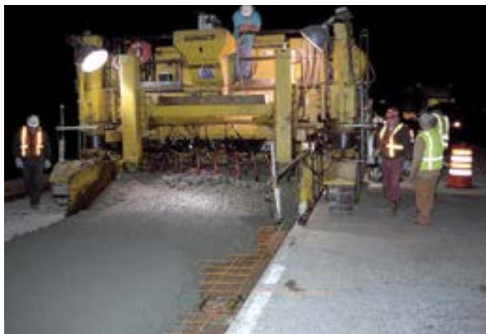
Figure 99. Controlling paving profile using a paver ski on the adjacent lane (source: Wouter Gulden, southeast chapter, ACPA)
