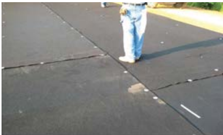
Figure 110. Overlap of nonwoven geotextile material section
