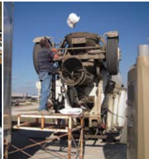
Figure 124. Fibers added at plant (left) and bags tossed into ready-mix truck (right) (source: Randell Riley, Illinois chapter, ACPA)
