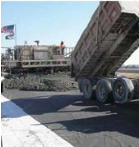
Figure 112. Paving on top of nonwoven geotextile materials
