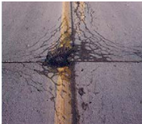
Figure 11. D-cracked pavement
