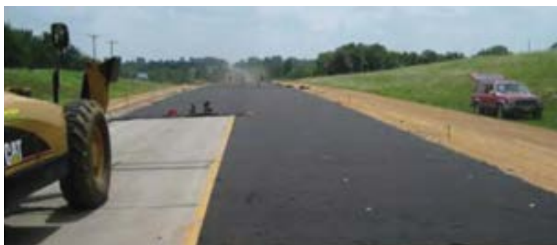
Figure 50. Geotextile fabric separation layer (source: Missouri DOT)
