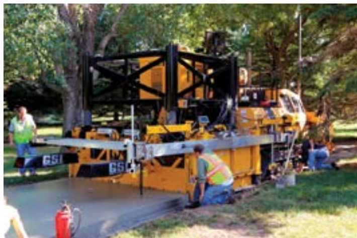
Figure 101. Zero clearance stringless paver (source: GOMACO)
