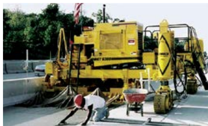
Figure 96. A three-track, zero-clearance paver placing concrete along a median barrier (source: Kevin Klein, Gomaco)
