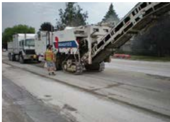
Figure 3. Milling concrete (left) and milled surface (right)
