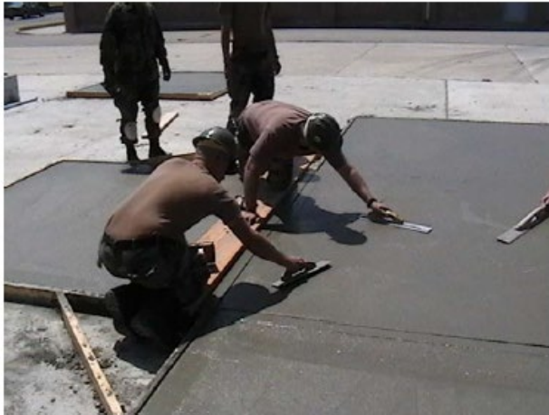
Figure 70 – Hand float in use.
