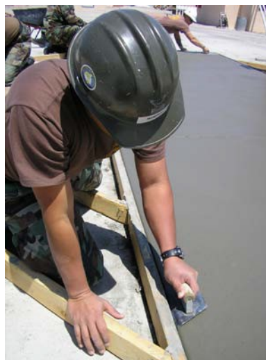
Figure 73 – Edger in use.
