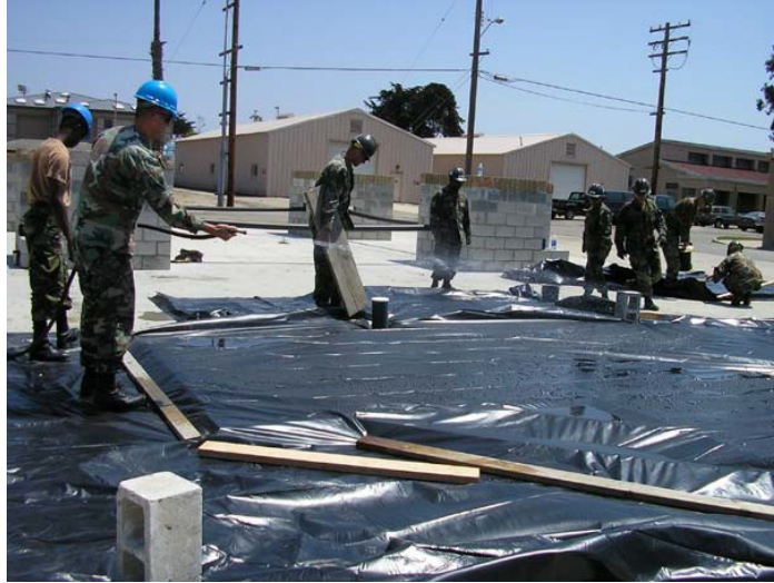
Figure 79 – Curing concrete with plastic.
