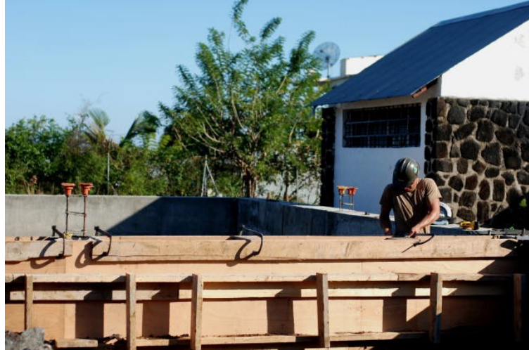
Figure 15 – Foundation forms.
