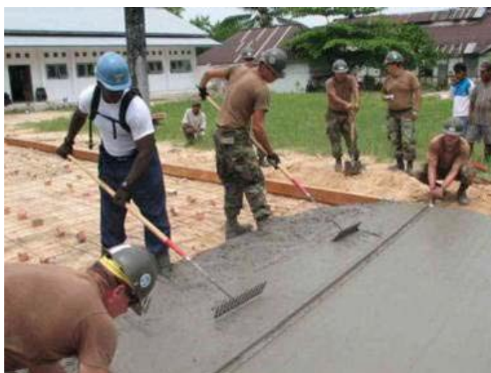
Figure 65 – Screeding operation.
