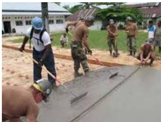
Figure 67 – Concrete placement.
