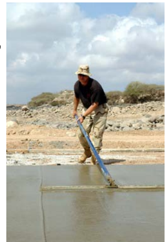
Figure 71 – Long handled float in use.
