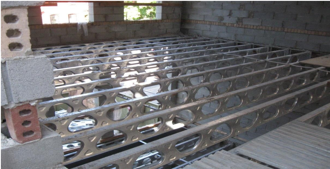
Fig. 6 Floor joists spaced at 16" o/c.
