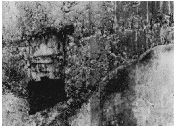
**Figure 2-2. Honeycombing and cold joint**
