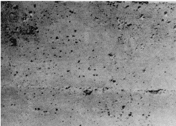
**Figure 2-1. Bug holes in a vertical wall**
