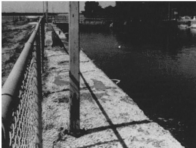
Figure 2-18. Severe scaling
