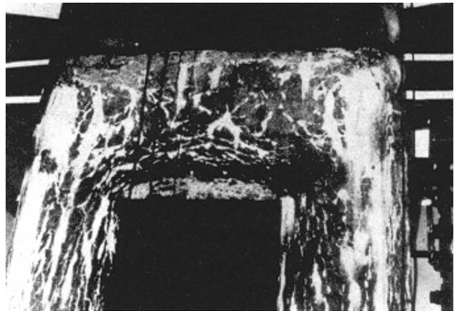
**Figure 2-24. Efflorescence**
