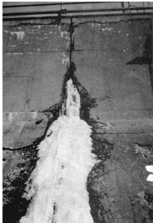
Figure 2-28. Water seepage through joint
