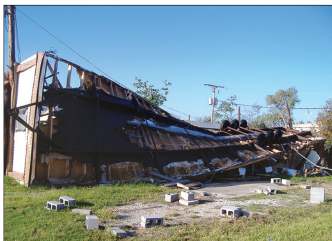
Figure 2-14. Manufactured home rolled over by Hurricane Katrina’s winds (Chalmette, Louisiana)
