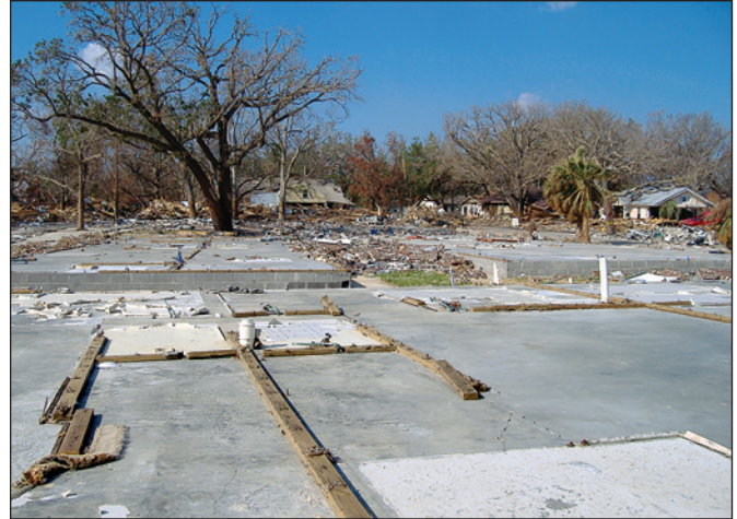
Figure 2-6. Waves, surge, and floating debris destroyed many single-family homes on slab foundations. Note the debris from houses that washed landward into other buildings (Biloxi, Mississippi).
