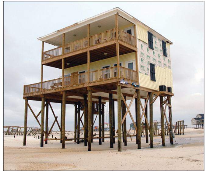
Figure 2-1. Successful example of well-elevated and embedded pile foundation following Katrina. Note adjacent building failures where foundations were not high enough or where pile embedment was insufficient (Dauphin Island, Alabama).
