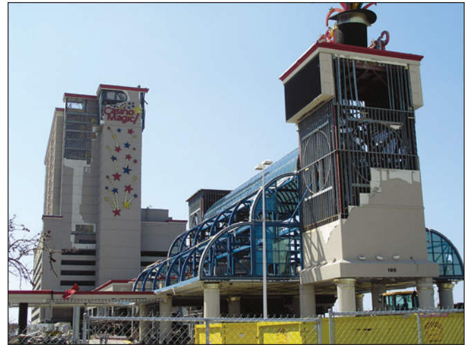
Figure 2-18. Multi-story building showing severe EIFS damage. In some areas, the gypsum board on the interior side of the studs was also blown away (Biloxi, Mississippi).
