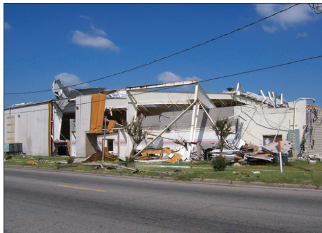
Figure 2-16. Pre-engineered metal building failure (Gulfport, Mississippi)
