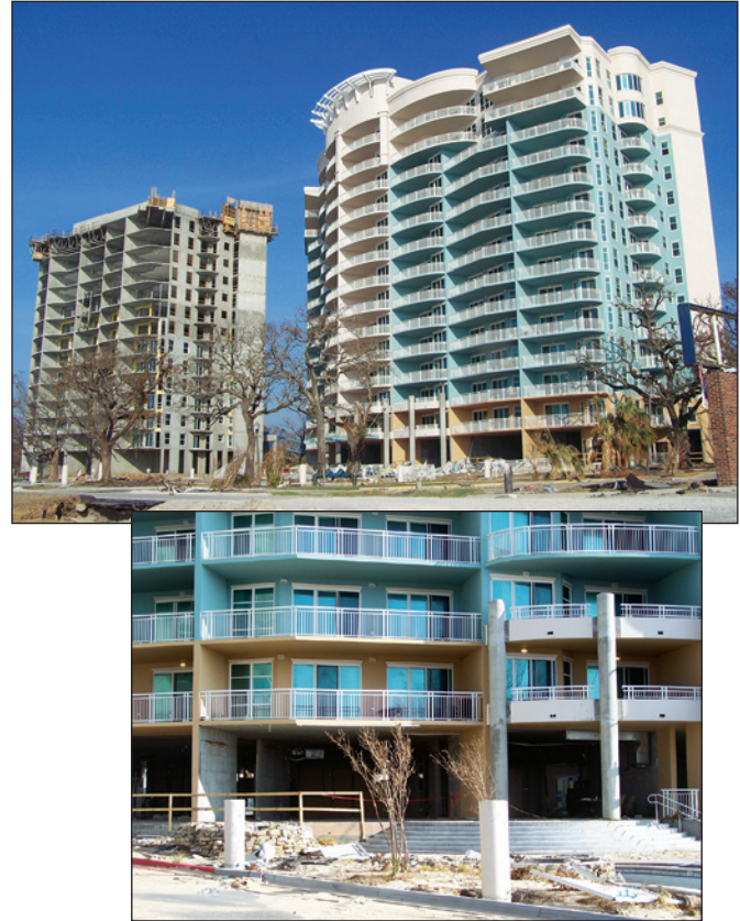
Figure 2-9. High-rise buildings along Beach Boulevard received non-structural flood damage to the lower floor, and no apparent flood or wind damage to higher residential floors (Gulfport, Mississippi)
