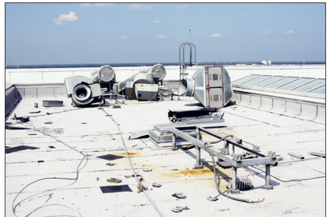
Figure 2-21. The equipment on this new Federal courthouse blew away because it was resting on vibration isolators that provided lateral resistance, but no uplift resistance. Two large openings through the roof were left after the ductwork blew away (temporary covers had been placed over the openings).
