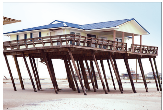
Figure 2-2. House that nearly failed due to insufficient pile embedment (Dauphin Island, Alabama)
