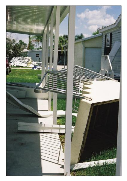
Figure 4-24. Stairway blown into a post of an aluminum carport accessory structure (Zolfo Springs)
