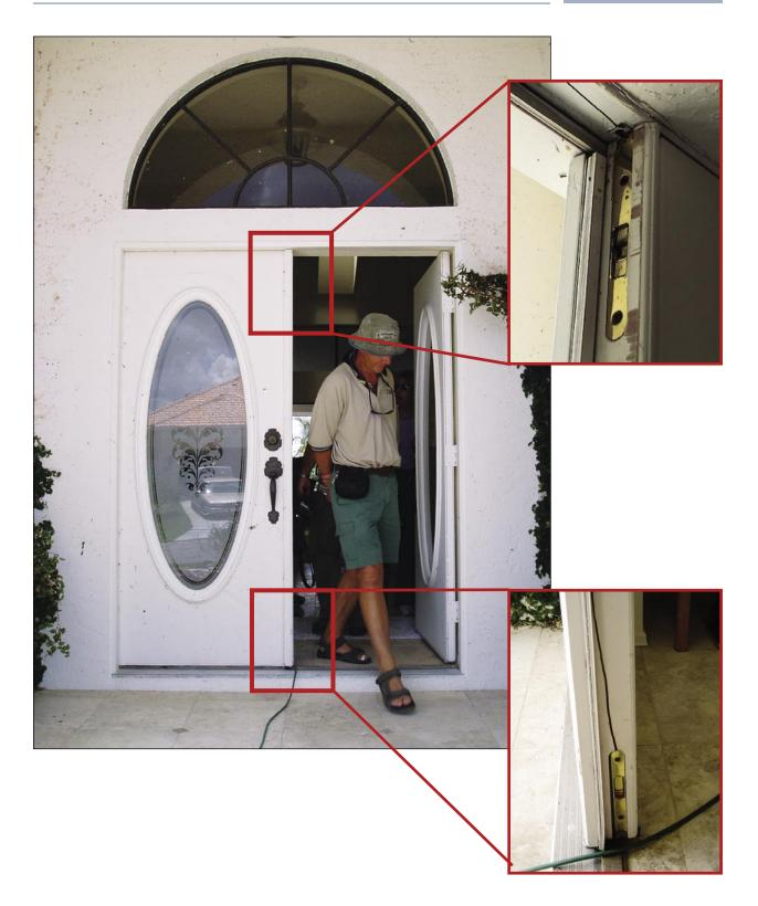
Figure 3-20. Double-entry door that failed under wind pressure. Upper inset shows close-up of crack in door frame at top latch. Lower inset shows crack in door emanating from bottom latch (Punta Gorda).
