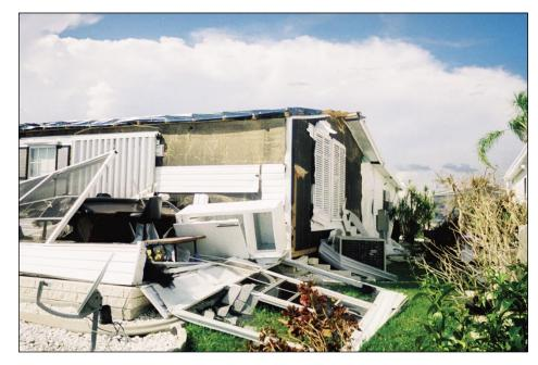
Figure 3-46. Example of damage to manufactured home roof covering, roof deck, and siding due to failure of screen enclosure attached to home (Port Charlotte)
