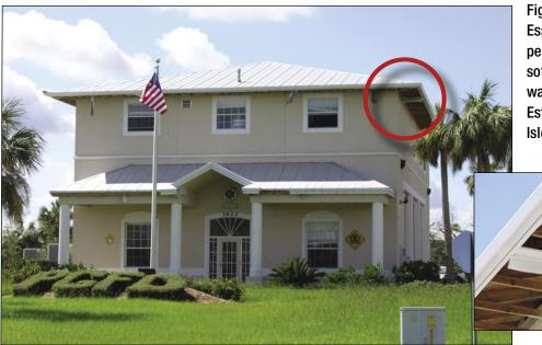
Figure 5-71. Essentially all of the perforated aluminum soffit on this fire station was blown away (Aqui Esta, east of Punta Gorda Isles).
