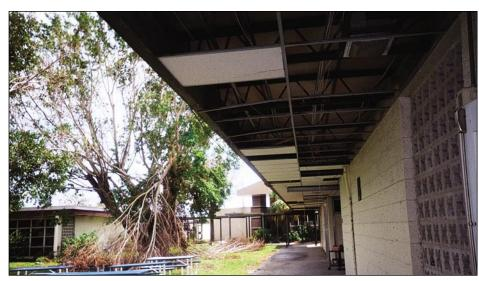
Figure 6-13. Loss of lightweight composite panel overhang at an elementary school (Charlotte Harbor)
