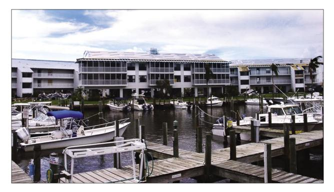
Figure 4-7. Multi-family residential building that performed well structurally, although it had severe roof covering and some sheathing failure at the overhangs, allowing water intrusion (Pine Island)
