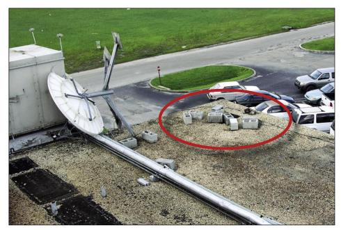
Figure 5-79. This satellite dish at a hospital was held down only with CMU. Note the loose LPS conductors and displaced air terminal at the corner (Arcadia).
