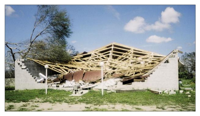
Figure 3-9. Example of wood truss roof failure due to sheathing loss and lack of bracing at gable end on a pre-2001 FBC unreinforced masonry building (north of Arcadia)
