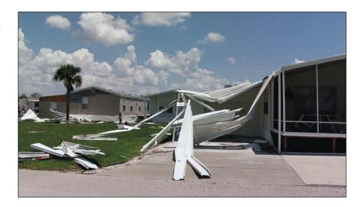
Figure 4-21. Damaged carport (Zolfo Springs)
