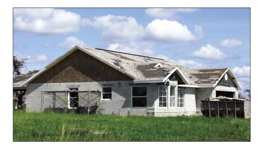
Figure 3-14. Asphalt shingle roof covering damage on a new one-story house. In some areas, the underlayment was also blown away (Deep Creek).
