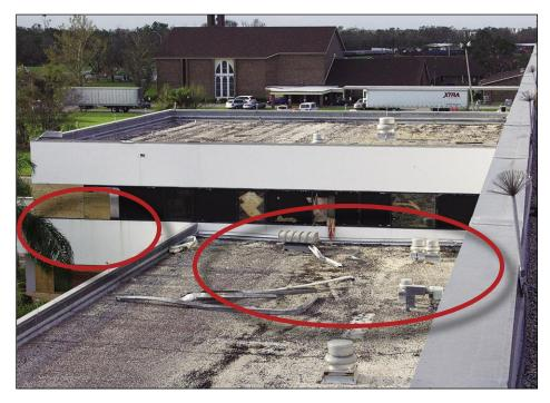
The gutters lying on the lower roof in Figure 6-8 came from the right side of the upper roof and may have caused some of the glass breakage. However, the majority of the damage was broken by flying aggregate from the hospital's BURs.
