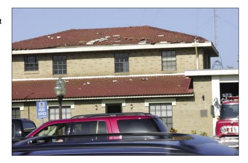
Figure 5-37. Fire station with at least three battens blown off. Some tiles remained attached (Fort Meade).
