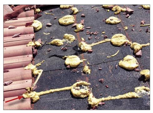
Figure 5-43. This photo clearly shows insufficient contact area of foam-set paddies on the bank's roof (Punta Gorda Isles).
