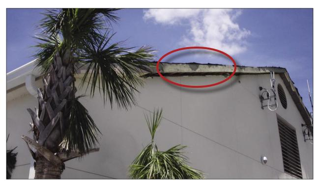
Figure 6-7. Damaged soffit at Punta Gorda Public Safety Complex
