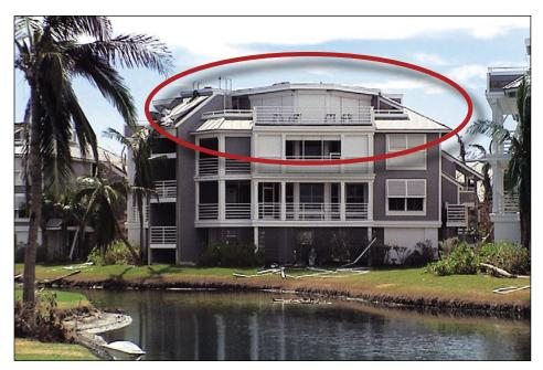
In addition to structural framing damage due to internal pressures, some wood buildings experienced failures due to a lack of continuous load path. Figure 3-5 is an example of a wood-frame structure that experienced a partial wall failure due to a lack of continuous load path. These types of damages were typically limited to areas along the path of the eye and were not typical of damage in areas with estimated wind speeds less than 100 mph (3-second peak gust).
