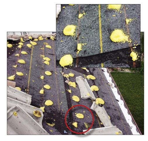
Figure 5-42. The paddy on the tile at the lower left debonded from the asphalt bleedout near a cap sheet lap. Only the center portion of the paddies made contact with the tiles, as shown in the inset (Punta Gorda Isles).
