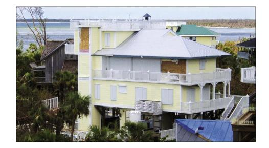
Figure 4-1. No structural damage was observed to new buildings built to the 2001 FBC standards (North Captiva Island).
