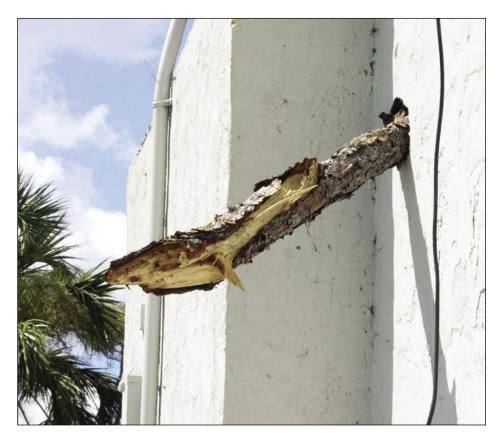
Figure 3-35. Impact of tree branch through the stucco and metal lath wall system of a fire station. The branch was about 5 inches in diameter and protruded about 3<sup>1</sup>/<sub>2</sub> feet out of the wall (Aqui Esta, east of Punta Gorda Isles).
