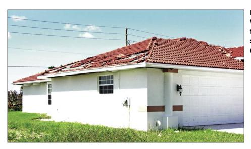
Figure 5-35. Windborne debris (likely tiles from this roof) broke several of the field tiles (Deep Creek).
