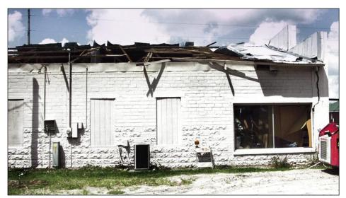
Figure 3-10. Roof sheathing and partial failure of wood roof structure on a masonry building. Note damage to inadequately reinforced masonry parapet at gable end wall (Wauchula).
