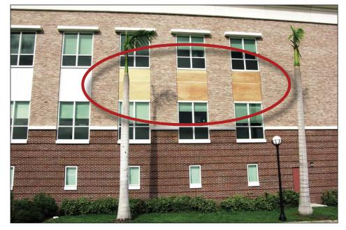
Figure 5-20. Plywood panels installed where aluminum spandrel panels were blown out of the curtain wall (Punta Gorda)
