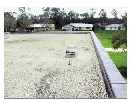
Figure 5-62. The edge flashing at this mineral surface cap sheet roof lifted (Port Charlotte).
