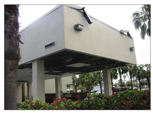
Figure 5-70. Loss of soffit at a bank drive-through. Note the coping damage (Port Charlotte).
