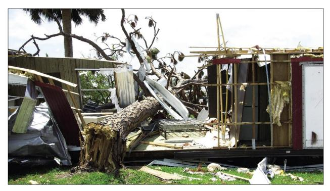
Figure 3-43. Damage to manufactured home from tree impact (Pine Island)
