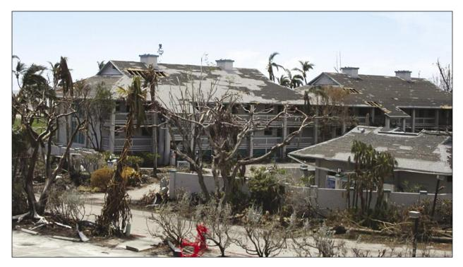
Figure 3-23. Roof covering loss. Note dark areas on roof are exposed underlayment (Captiva Island).
