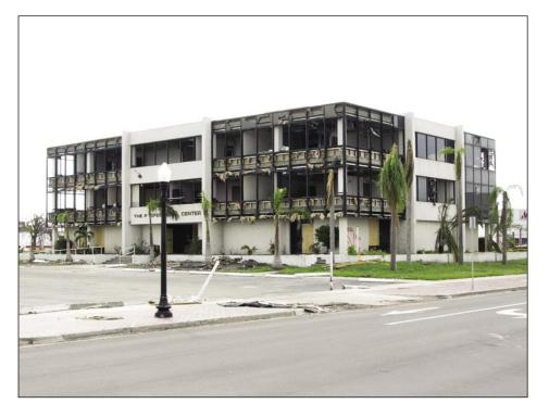
Figure 5-19. Windows broken by aggregate from a nearby BUR. Besides impact at the crack intersection, aggregate chipped the glass in three other locations (Punta Gorda).
