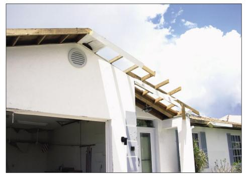
Figure 4-6. Roof decking failed due to uplift (Deep Creek)
