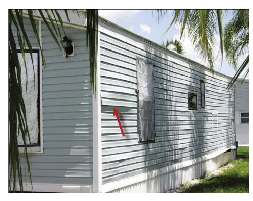
Figure 5-65. The vinyl siding panel with the red arrow is unlatched. The panel above and several others are also unlatched (Zolfo Springs).
