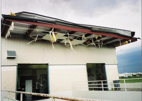
Figure 6-3. Failure of roof and soffit panels at rear awning (Charlotte County EOC)
