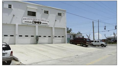
Figure 3-54. Fire station elevated on fill prevented any storm surge damage (Fort Myers Beach)
