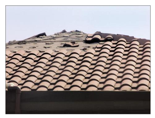
Figure 5-32. Most of the mortar-set hip and ridge tiles blew off this house (Port Charlotte).
