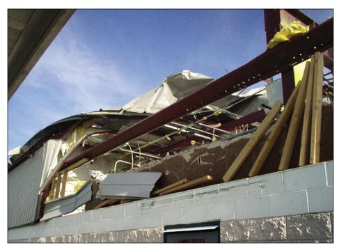
Wind induced wall damage was limited to the upper portions of the exterior walls constructed of metal panels attached to the steel frame and to wood studs acting as purlins between the frame and the top of the masonry walls. Failures observed varied from clip and connection failures, similar to those observed with the roof panels, to complete failures of stud-supported sections (Figure 6-3).
