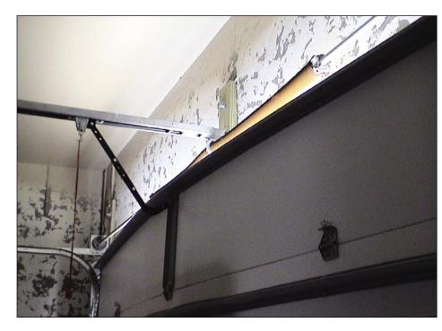
Figure 5-6. Garage door failed because the removable stiffener bar was not in place at the time of the hurricane (Punta Gorda Isles).
