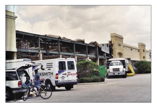
Figure 4-16. Older steel-frame structure performed well in spite of major damage to the roof decking and the exterior walls (Wauchula)
