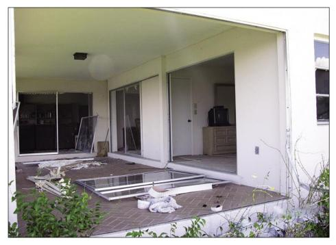
Figure 5-1. Sliding glass doors blown out of their tracks (Punta Gorda Isles)
