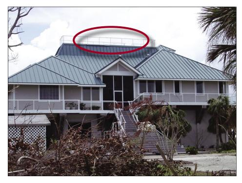
Figure 7-1. Residence constructed to the design requirements of the 2001 FBC performed well and only experienced some light trim damage (shown in the center of the photo) (North Captiva Island).
