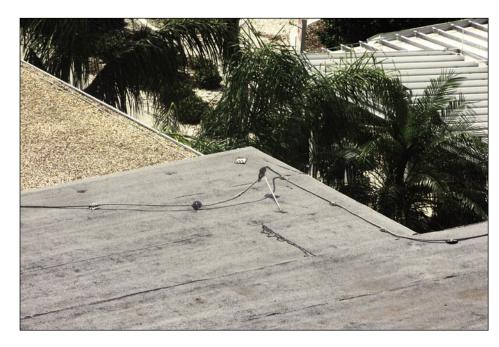
Figure 5-83. The conductor connectors detached from the cap sheet on a hospital's BUR. The air terminal was also displaced (Port Charlotte).
