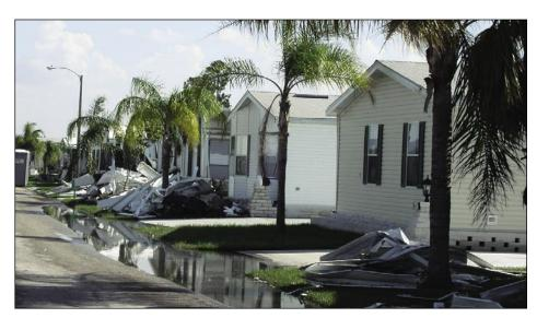
Figure 3-39. Typical metal roof panel and siding debris from failed accessory structures and manufactured homes that were stripped of siding resulting from accessory structures failure (Arcadia)
