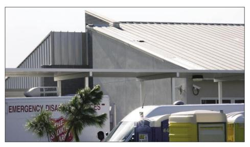
Figure 5-56. Several of the architectural panels and hip flashings blew off this fire station (Deep Creek).
