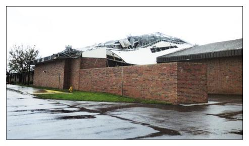
Figure 6-12. Collapsed gable end wall at an elementary school (Deep Creek)
