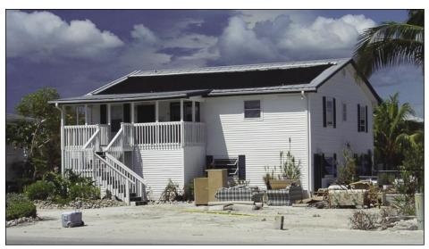
Figure 3-52. Typical house with firstfloor living space at grade sustained 2 to 3 feet of storm surge damage (lack of wall damage suggests low velocity flows) (Fort Myers Beach)
