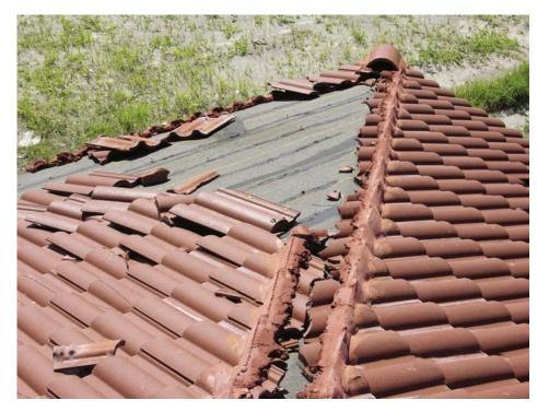
Figure 5-36. Loss of mortar-set hip tiles and several of the field tiles. Some of the screws remained in the deck, while others had been pulled out (Deep Creek).
