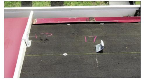
Several structural standing-seam trapezoidal panel system failures were observed, including the panels on the Turner Agri-Civic Center in Arcadia, which partially collapsed (see Section 6.5.1.1. and Figures 6-17 and 6-18). It was reported that the roof covering was lifting prior to the collapse. The panels were installed over fiberglass batts over a vapor retarder atop the light-gauge purlins.
