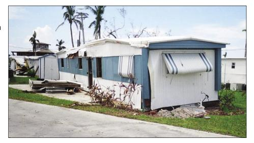
Figure 3-8 experienced extensive structural damage from 3-second peak gust winds in excess of the range of 110 to 130 mph.
