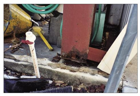
Figure 4-20. Significant amount of corrosion at Fire Station No. 8, which contributed to failure shown in Figure 4-19
