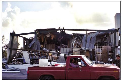
Figure 4-17. Completely destroyed pre-engineered metal building (Arcadia)
