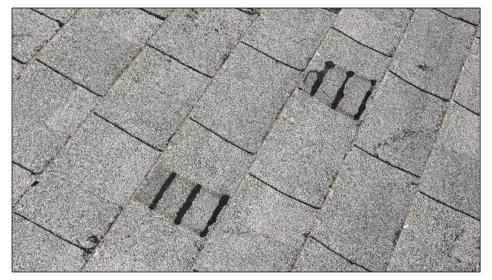
Figure 5-27. Two laminated tabs blown off (Deep Creek)
