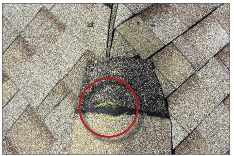
Figure 5-26. Only the portion of the self-seal adhesive that is indicated in yellow had bonded (within the red circle). No bonding occurred on the right side of the hip line (Deep Creek).
