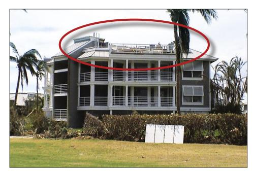
Figure 3-4. Nearby undamaged wood-frame building similar to that shown in Figure 3-3 protected with shutters (Captiva Island)
