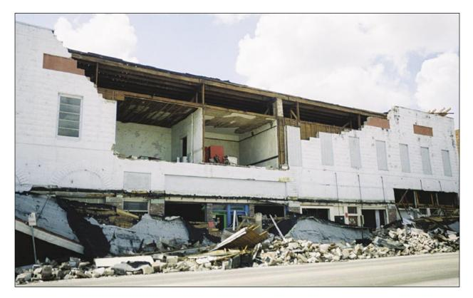
Figure 3-25. Example of unreinforced masonry wall and parapet collapse due to breaching of roof (on opposite side of building) (Wauchula)
