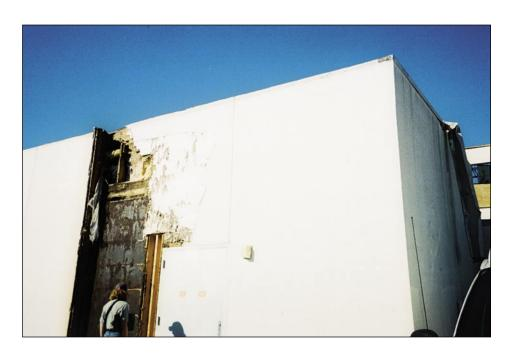
Damage to windows, doors, and soffits was observed in commercial applications similar to the losses and damages observed in residential construction. Figure 3-27 is a medical office building in Punta Gorda that lost roof decking, suffered damage to EIFS wall coverings, and experienced significant glass breakage.
