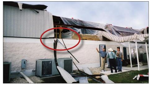
Figure 6-1. Exterior wall and roof damage at Charlotte County EOC
