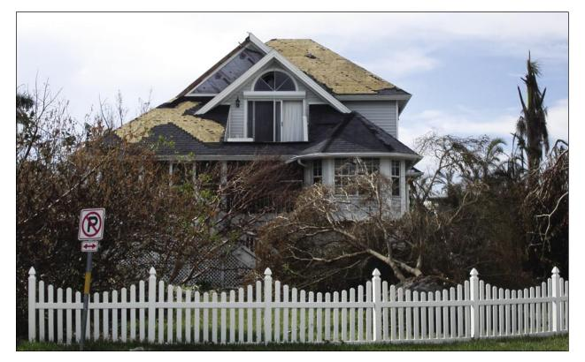
Figure 3-15. Typical asphalt shingle roof covering loss on elevated, two-story house (Captiva Island)
