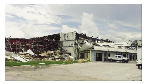
Figure 3-12. Pre-engineered metal building with progressive failure and severe panel loss (Arcadia)
