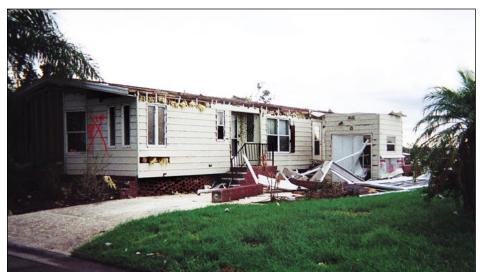
Figure 3-45. Example of typical damage to roof covering, roof sheathing, and exterior siding of a manufactured home as a result of the failure of an attached carport structure (Port Charlotte)
