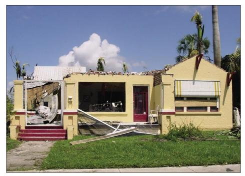
Figure 3-2. Failure of roof structure from pressurization of a pre-2001 FBC house when the window failed on windward face (Punta Gorda)
