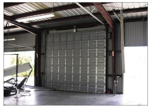
Figure 5-9. Windward side of a fire station; two doors blew inward, but the newer center door remained intact (Punta Gorda).
