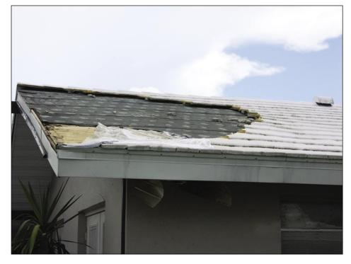
Figure 5-47. The other side of the roof shown in Figure 5-46 with a portion of the underlayment and several tiles blown off (Punta Gorda Isles)
