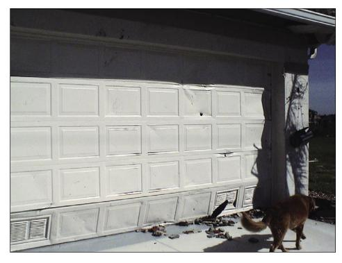
Figure 3-36. Tile damage to a metalpanel garage door (Punta Gorda)
