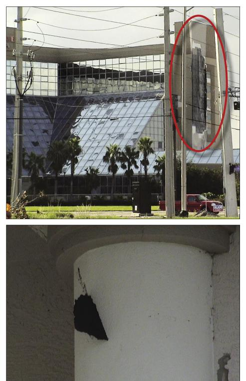
Figure 3-34. Edge impact of an asphalt shingle on decorative column (Punta Gorda)
