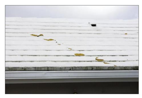
Figure 5-46. This residence had a tile roof that had been covered with SPF. A missile gouged the foam, but no tile debris was blown off (Punta Gorda Isles).
