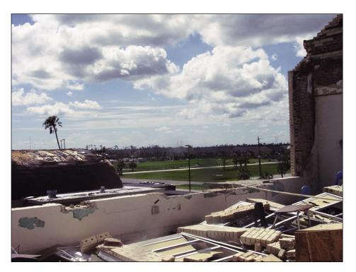
Figure 4-13. Unreinforced brick wall failure of a building built over 50 years ago (photo taken from the inside of a classroom, looking out) (Punta Gorda)
