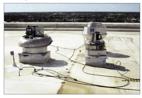
Figure 5-76. Cowlings blown off two exhaust fans in the foreground. Note also the loose LPS conductors and missing walkway pad (Punta Gorda). Loss of HVAC units was also observed as shown in Figure 5-77. A number of these large units were blown off their supports. Additional damage to equipment included loss of access panels on package units, debris impact damage to relief air hoods, and damaged rooftop ductwork. Figure 5-78 shows a unit that was marginally anchored.
