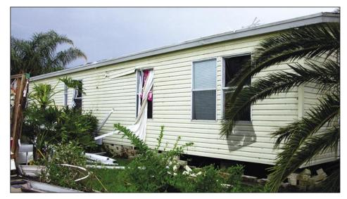
Figure 5-11. Most of the windows on this side of a manufactured home were broken by windborne debris (east of Port Charlotte).
