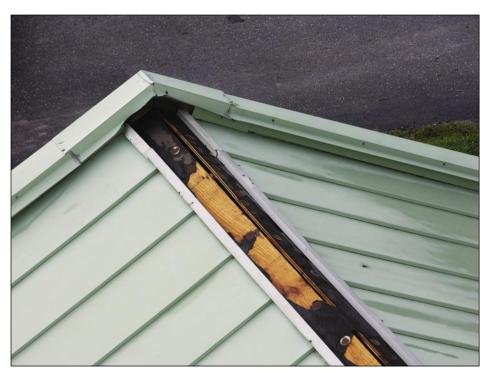
Figure 5-54. View of the canopy ridge at the building shown in Figure 5-52. The ridge flashing fasteners were placed too far apart. A significant amount of water leakage can occur when ridge flashings are blown away (Port Charlotte).
