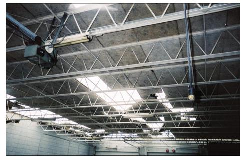
Figure 3-56. Cementitious wood-fiber roof deck panels at this older fire station were not adequately secured to resist uplift (Port Charlotte).
