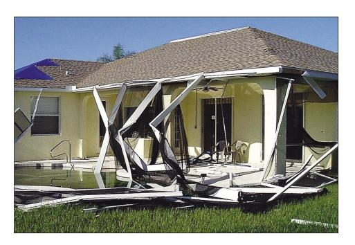
Figure 4-26. Consequence of corner post not directly tied down to the slab (Punta Gorda Isles)
