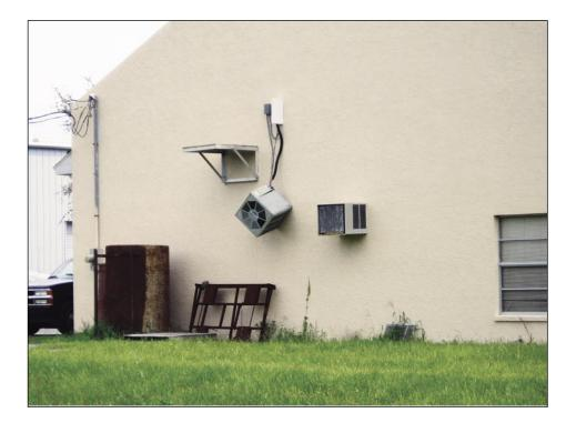
Figure 5-74. Condenser unit displaced from the elevated platform (Port Charlotte)
