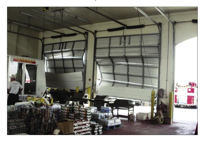
Figure 3-28. Damage to large rolling and sectional doors at Fire Station No. 1 (Punta Gorda)
