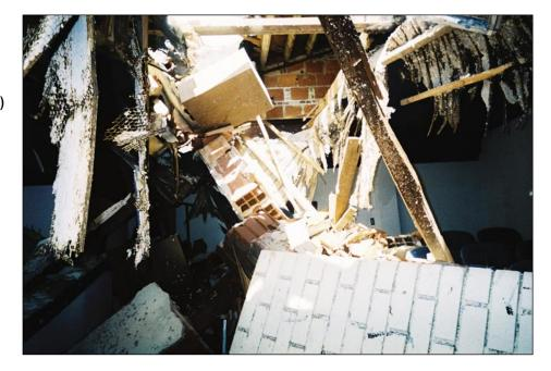
Figure 6-11. URM parapet damage to front façade of a high school (Punta Gorda)
