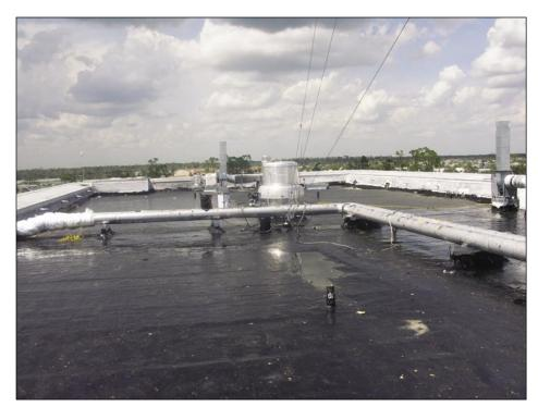
Figure 5-64. View of a portion of the fourth floor roof of a hospital after installation of an emergency roof (the black area). The deck was concrete (Port Charlotte).
