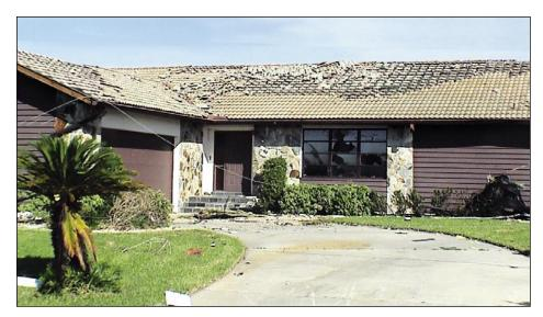
Figure 3-31. Extensive damage to mortar-set tile roof on this pre-2001 FBC home. Note broken windows to the right of the front door (Punta Gorda).
