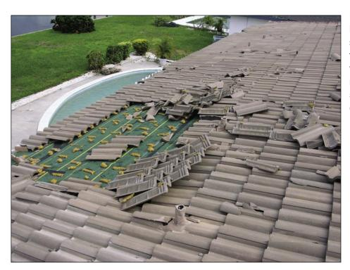
Figure 5-38. In addition to the damage shown in this photo, this one-story roof lost virtually all of the hip and ridge tiles (see Figures 5-22, 5-39, and 5-40) (Punta Gorda Isles).
