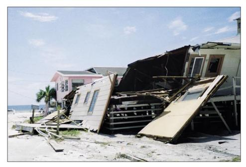
Figure 3-5. Wall failure on older multi-family wood-frame building due to lack of continuous load path. Internal pressurization may have also contributed to this failure (Fort Myers Beach).
