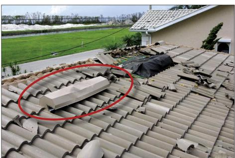
Figure 5-22. The attic vent to the right (temporarily covered with felt) on this foamset tile roof lifted during the hurricane and allowed water to enter the residence shown in Figure 5-21. The failed vent is like the one on the left (Punta Gorda Isles).
