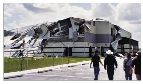
Figure 6-18. End wall failure at Turner Agri-Civic Center (Arcadia)
