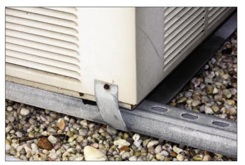
Figure 5-75. Rooftop condenser anchored to a support rail, but with only one small screw (which was corroded) used to connect the strap (Port Charlotte).
