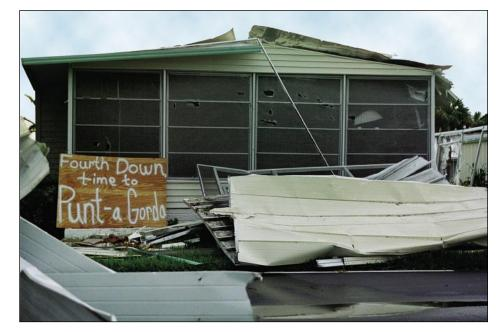
Figure 4-23. Damaged screened porch (Punta Gorda)
