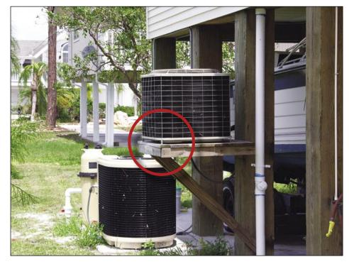
Figure 5-73. Condenser on the elevated platform attached with four angle brackets. The other condenser, located adjacent to it on the ground, should also have been on an elevated platform to account for storm surge (Pine Island).
