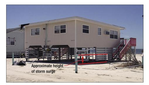
Figure 3-51. Storm surge damage of 2 to 3 feet limited to lower floor of two-story house
