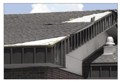
Figure 5-29. Edge flashing that caused a progressive failure of the shingles (Deep Creek)
