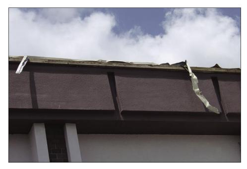
Figure 6-22. Edge flashing failure at Port Charlotte Middle School
