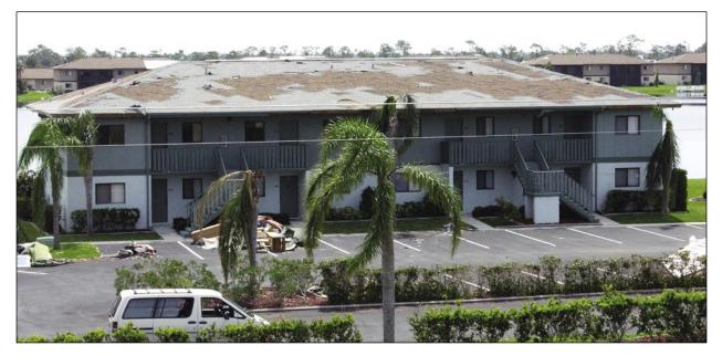
Figure 5-28. Re-covered apartment building (the newer shingles are grey and the older shingles are brown) (Deep Creek).
