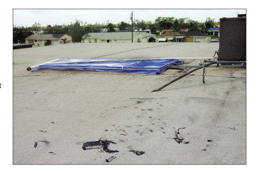
Figure 5-77. A large HVAC unit blew off this curb. Note the loose LPS conductors (this side of the curb). This school had significant damage to several pieces of rooftop equipment (Port Charlotte).
