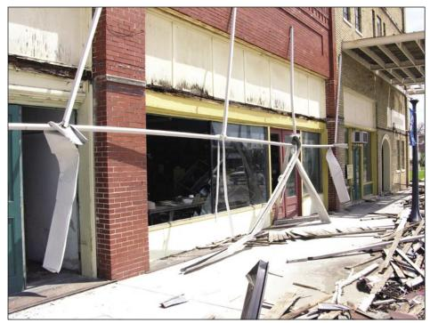
Figure 5-18. All of the glazing, including glass spandrel panels, was broken on the long side of the building (Punta Gorda).
