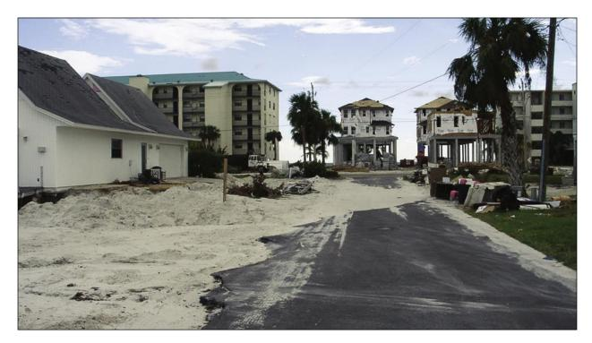
Figure 3-55. Storm surge caused scouring of the road and damage to the infrastructure (i.e., water main) (Fort Myers Beach)
