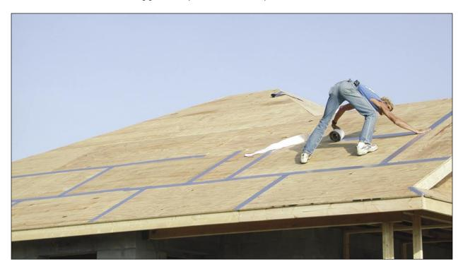
Figure 5-23. Installation of self-adhering modified bitumen tape at sheathing joints, as part of an enhanced underlayment system on a Fortified...for safer living<sup>™</sup> house under construction (IBHS)
