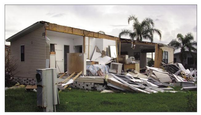
Figure 3-8. Post-1994 manufactured home with major roof and wall failure (east of Port Charlotte)
