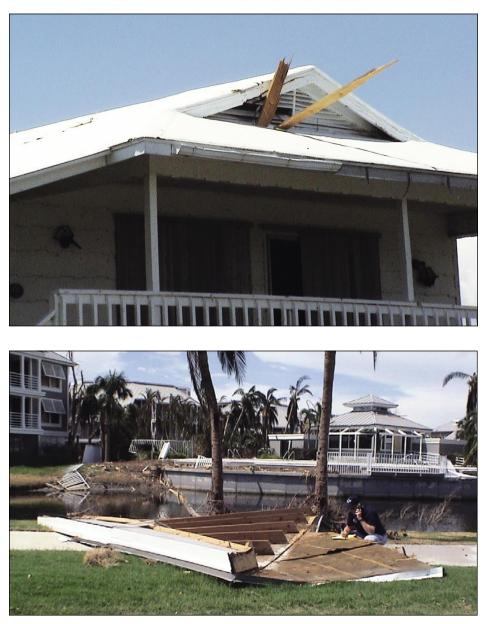
Figure 3-38. Large section of roof structure transported over 200 yards from its source (Captiva Island)
