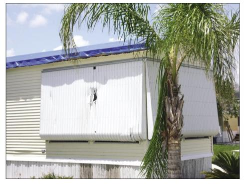
Figure 5-14. Metal awning shutter penetrated by a missile (Zolfo Springs)
