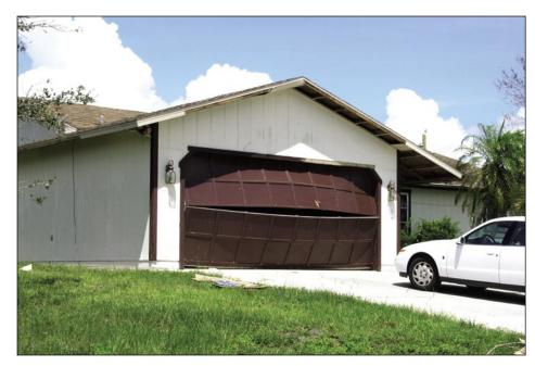
Figure 5-4. Door lacked sufficient strength to resist the suction load (Deep Creek)
