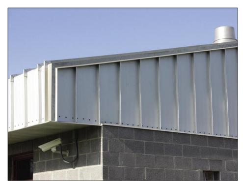
Figure 5-67. Standing seam metal panels with a 16-inch rib spacing were used at the fascia and secured with closely spaced exposed fasteners (Arcadia).
