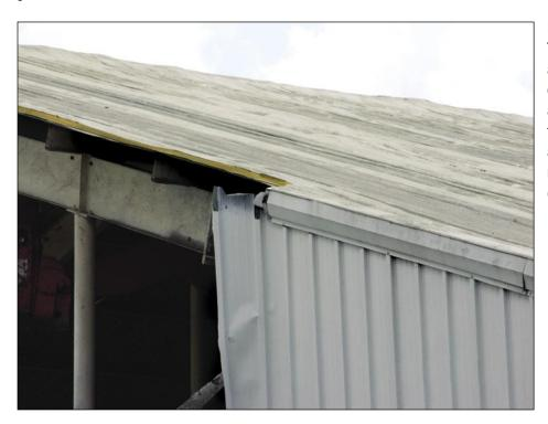
Figure 5-58. The metal wall panels and metal edge flashing on this building blew away, but the exposed fastener R-panels with an SPF covering did not progressively fail (Wauchula).
