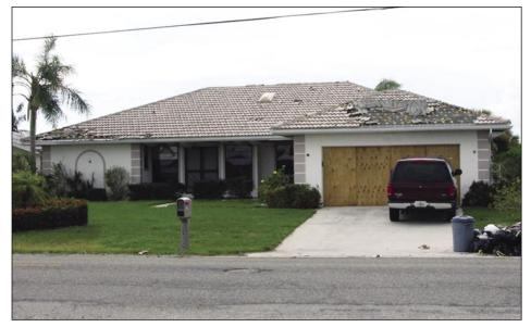
Figure 5-41. In addition to field tile blow-off, most of the hip tiles and several ridge tiles were also blown off this house (Punta Gorda Isles).
