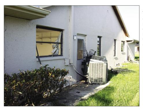
Figure 5-72. This condenser was not anchored to the concrete pad. The electrical and copper tube connections kept it from blowing farther away (Deep Creek).
