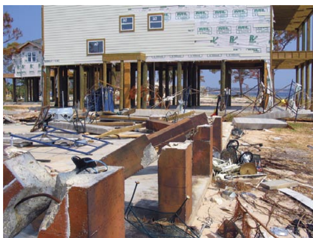
High flood levels during Hurricane Ivan and lack of structural capacity to withstand waves and debris loads caused this reinforced pier foundation to fail.
