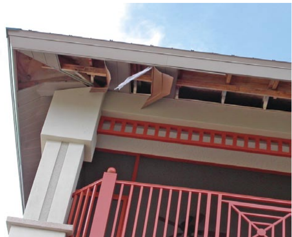
Soffit damage on the third story of a multi-family building. (Captive Island)
