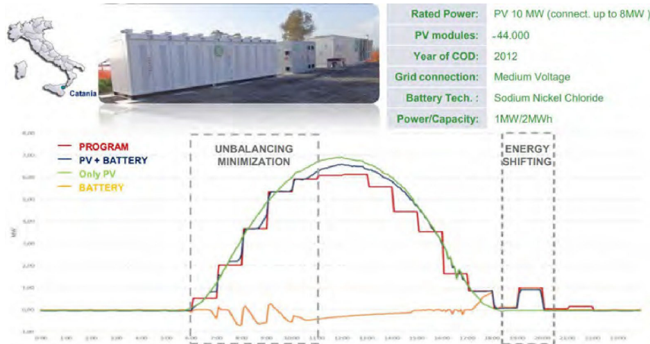
Figure 3.5: Solar Photovoltaic Installation with a Storage System
