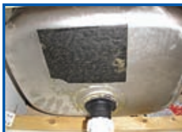
Chrysotile-containing bitumen pad to underside of sink
