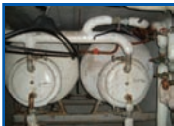
Thermal insulation to calorifier
