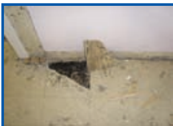
Chrysotile-based floor tiles and chrysotile containing adhesive
