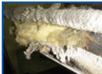
Chrysotile rope lagging to pipework
