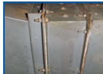
Chrysotile rope seals to flanges of ductwork
