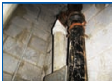
Asbestos cement flue pipe
