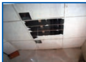
Damaged AIB ceiling panels
