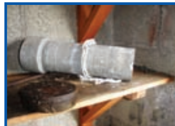
Chrysotile rope to asbestos cement flue pipe
