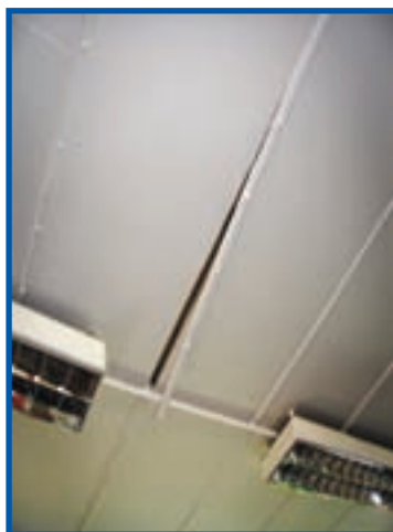
Asbestos cement ceiling panels
