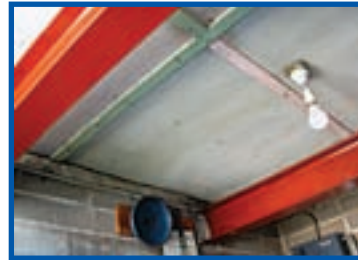
AIB ceiling panels in lift motor room
