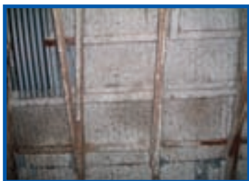
Asbestos spray coating to metal corrugated roof
