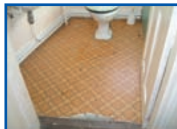
Chrysotile backing to linoleum floor covering
