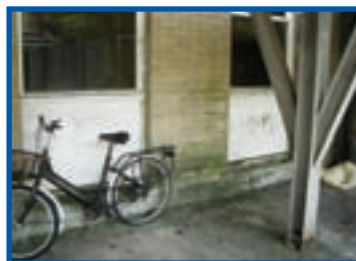
Asbestos cement wall panels
