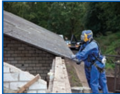
Asbestos worker incorrectly wearing full face respirator (head straps outside hood). The worker must remove his respirator to allow him to remove his contaminated overalls which is poor practice.
