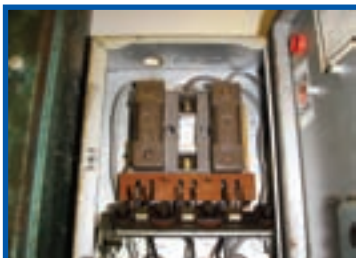
Chrysotile flash guards in old fuse box
