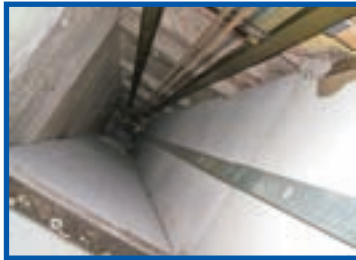
AIB lining to dumb waiter shaft
