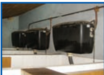
Asbestos-containing shires lynx toilet cisterns
