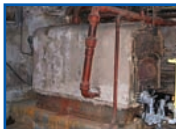
Thermal insulation to boiler
