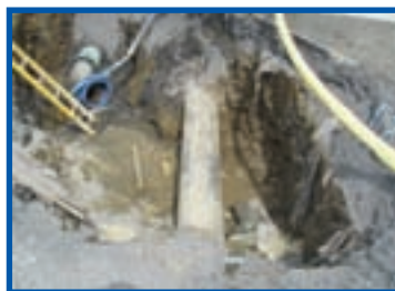
Asbestos cement water main
