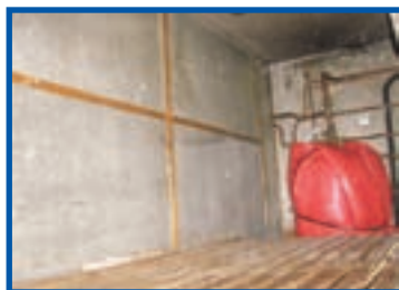
Asbestos cement wall panels in hot press
