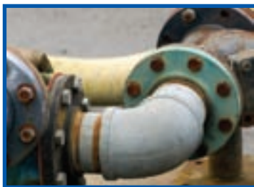
Compressed asbestos gaskets to pipework flanges
