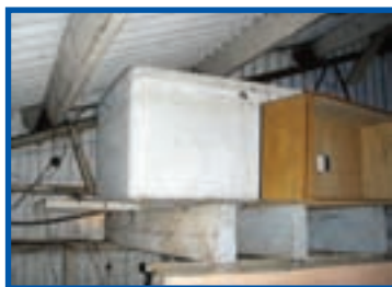
Asbestos cement water tank in attic
