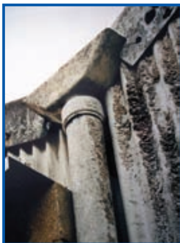
Asbestos cement barge boards and downpipe
