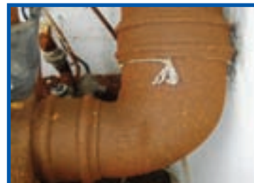
Chrysotile rope to metal to boiler flue
