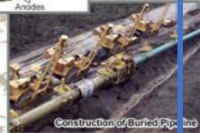
Construction of Buried Pipeline
