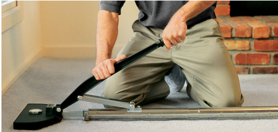
Figure 2.13 stretch-in installation
