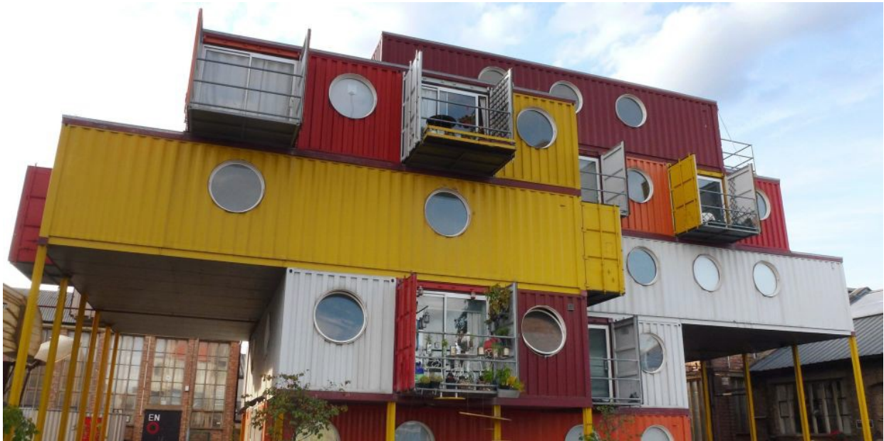
Figure 3.18 Technically advanced modular steel installation: The modules can be stacked vertically and horizontally on one another. The floor area can be therefore reduced or increased based on the required program. (Source: Source:www.designingbuildings.co.uk 2100 × 1481)
