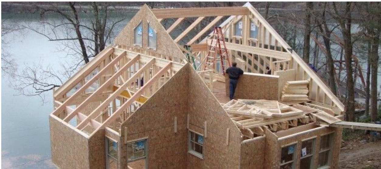
Figure 3.1 Installation of a panelized wooden wall. (Source: Logangate Timber Homes)
