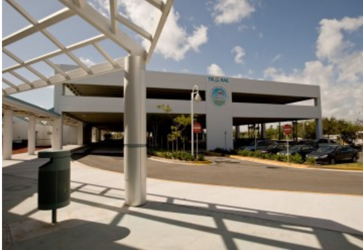
Figure 3.38 Dania Beach Park-N-Ride Parking Garage, Dania Beach, Florida. This garage, completed in 2010 by FINFROCK, serves passengers for the Tri-Rail high-speed rail line that serves Broward, Miami-Dade, and Palm Beach Counties. It has 402 stalls, and two stories. (Source: Finrock)
