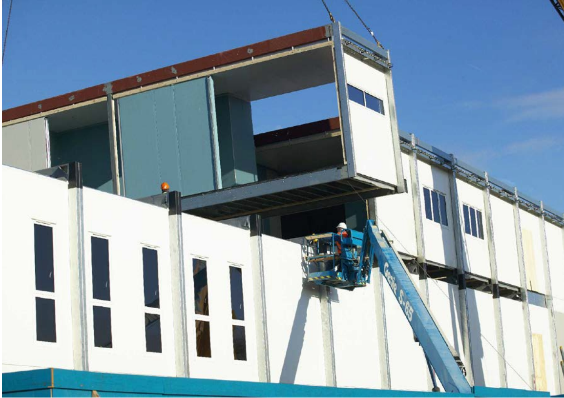
Figure 3.18 Technically advanced modular steel installation: The modules can be stacked vertically and horizontally on one another. The floor area can be therefore reduced or increased based on the required program. (Source: Source:www.designingbuildings.co.uk 2100 × 1481)
