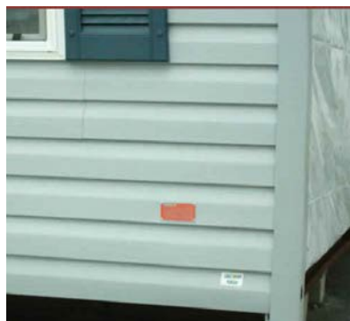
Figure 1.5 The Certification Label must be permanently attached to every manufactured home sold in the U.S.
