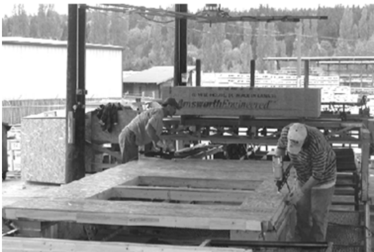
Figure 3.3 Application of sheathing panels to framing. (Source: U.S. Department of Housing and Urban Development)
