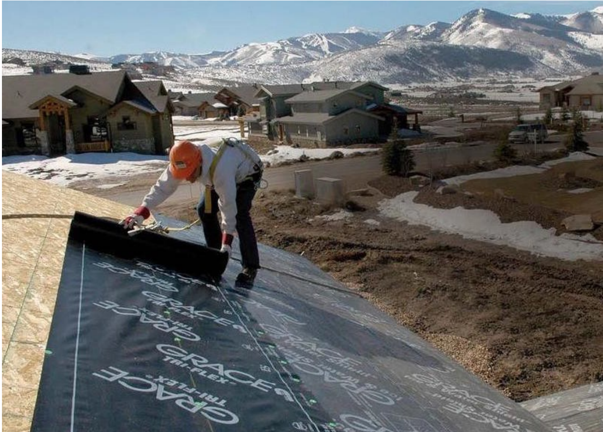
Figure 2.3 Asphalt felt roll installation
