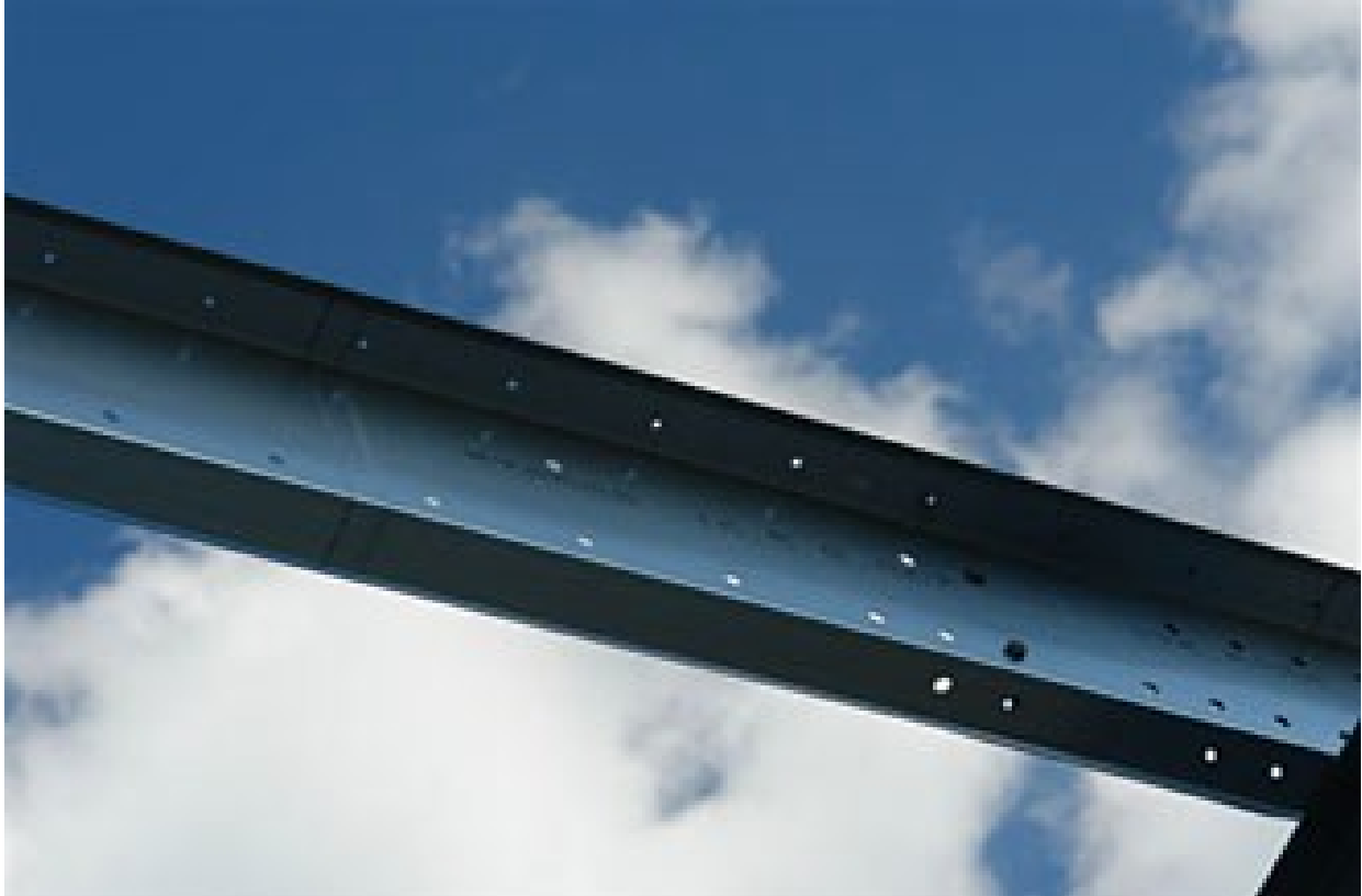
Figure 3.21 Punching the steel members in the factory creates a perfect alignment facilitating correct alignment. The holes are not only used to attach the primary framing together but to create a seamless and weather-proof shell. Especially in roof planning, proper alignment of roof panels is crucial to short and long term roof performance. Poor alignment affects weather-tightness and creates problems when installing closures, roof accessories, and trim. (Source: Butler Manufacturing)
