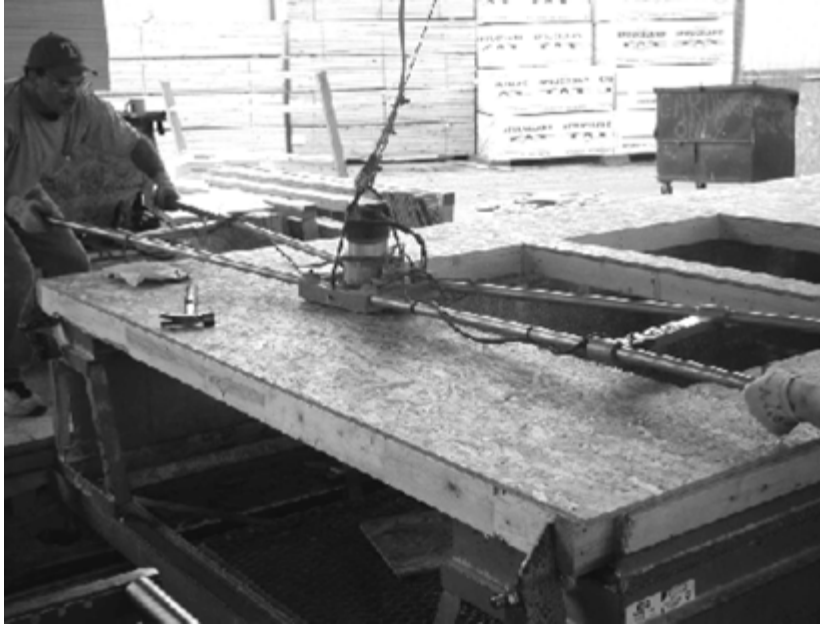
Figure 3.4 A router is used to create panel openings. (Source: U.S. Department of Housing and Urban Development)
