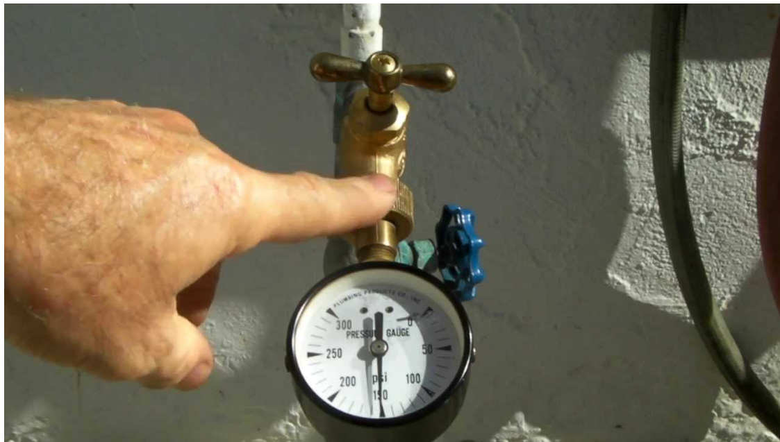
Figure 2.34 Water pressure test
