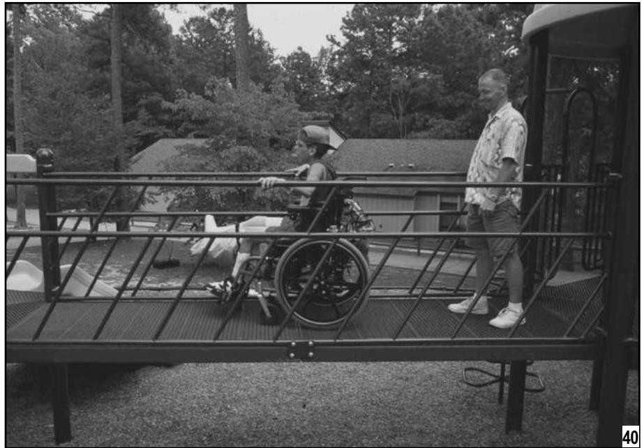
This photo illustrates an elevated accessible route:
