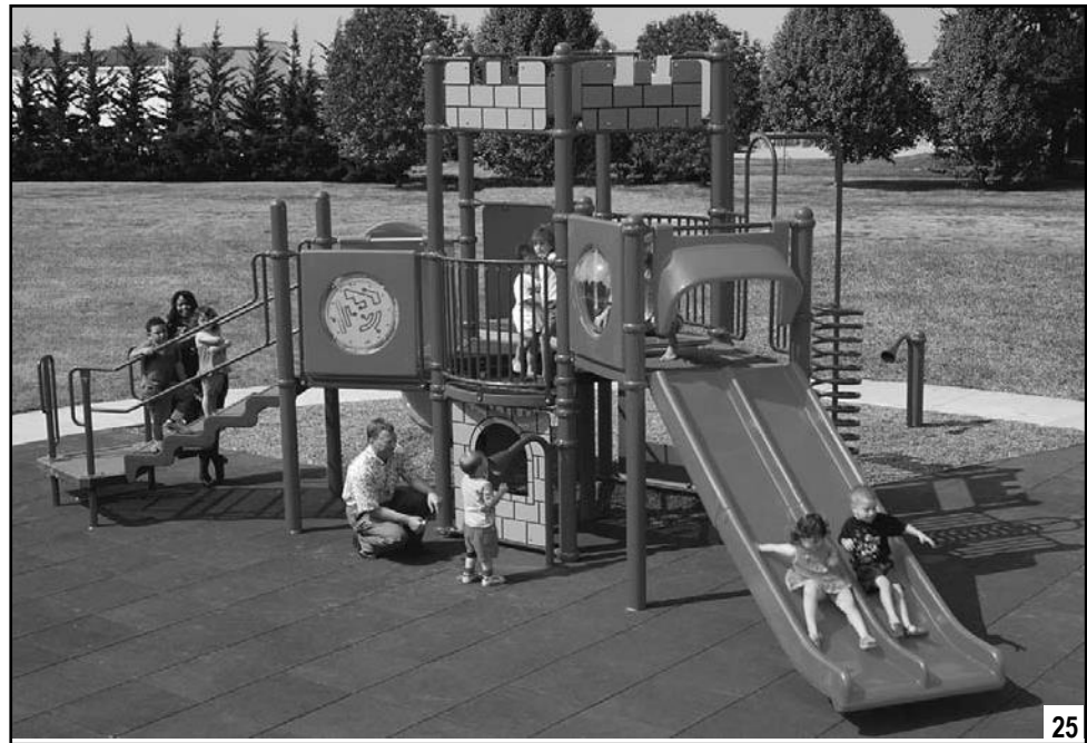
Play areas with less than 20 elevated play components may use a transfer system instead of ramps to connect at least 50 percent of the elevated components.
