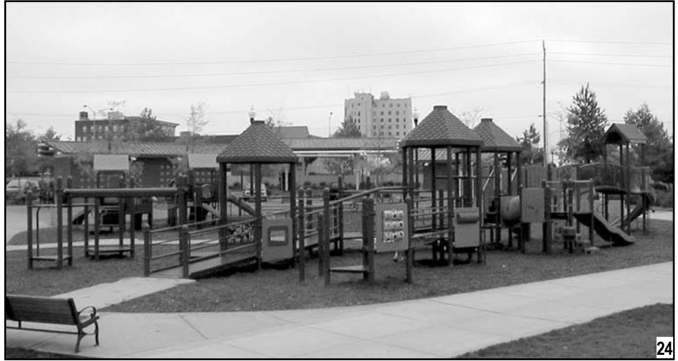
Play areas with 20 or more elevated components must use ramps to connect a minimum of 25 percent of those components. A transfer system or ramps may connect the other elevated play components required on an accessible route.
