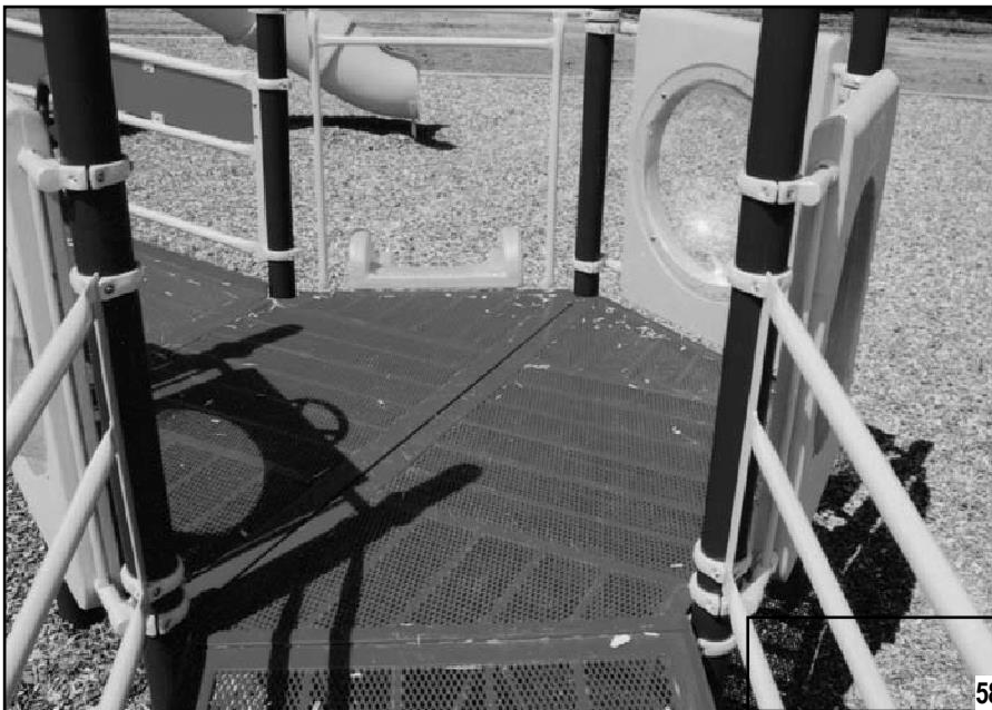
The clear floor space is permitted to overlap onto the landing area to provide access to this elevated window activity.
