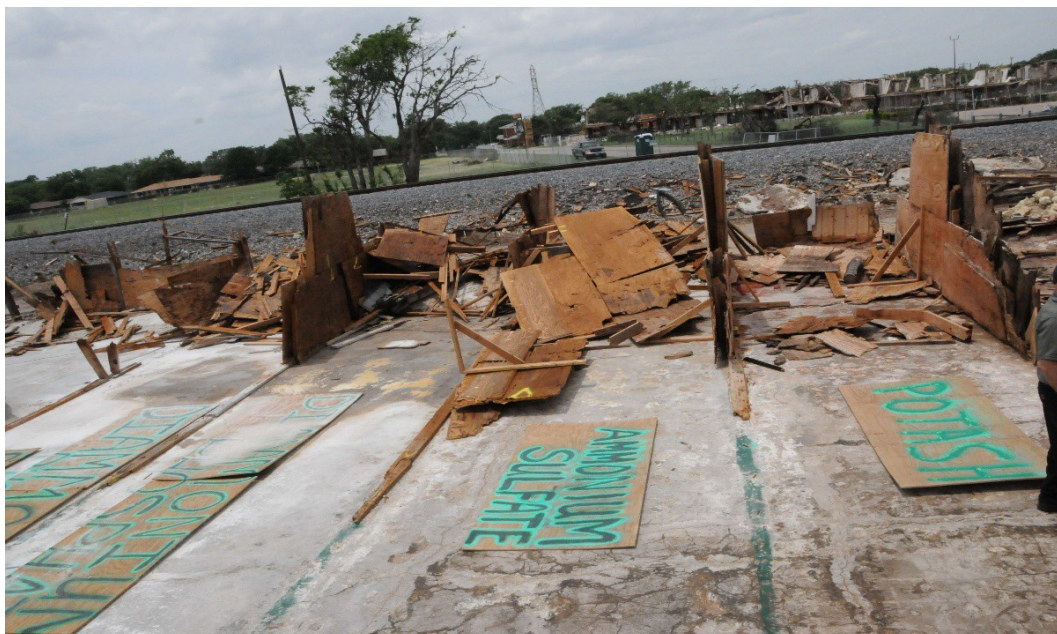
Figure 8. Plywood Bin Wall, Post-Explosion (Source: CSB)
