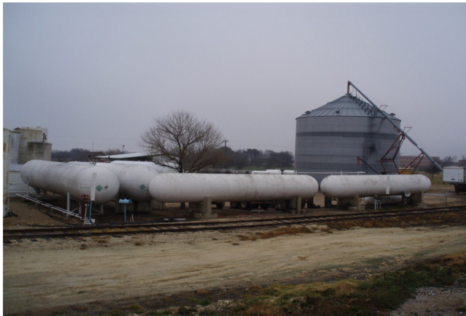
Figure 6. Anhydrous Ammonia Storage (Source: WFC Insurer)
