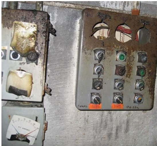
Figure 22. Non-dust rated and rated electrical devices in the silo tunnel
