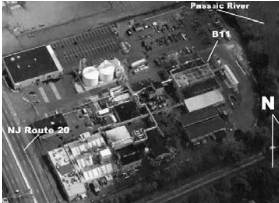
Figure 1: Aerial View of the Paterson Plant
