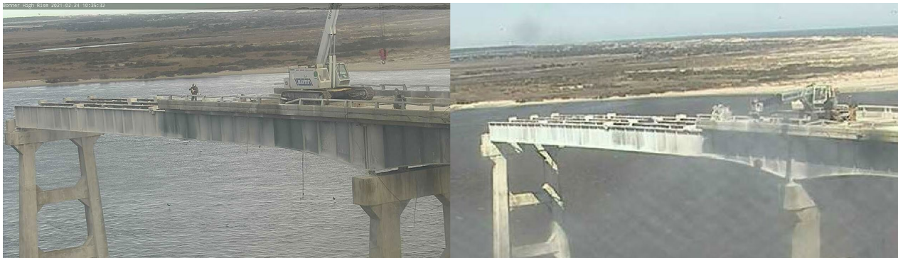
Demolition progress on 2/24/2021
