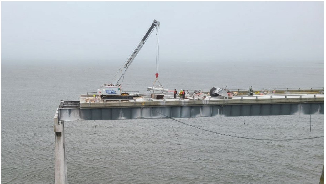
Figure 13 – Demolition of Span 144 (photographed on 2/15/2021 by NCDOT)
