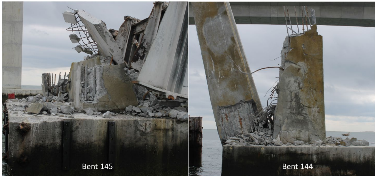
Figure 30 – Collapsed Bent 144/145
