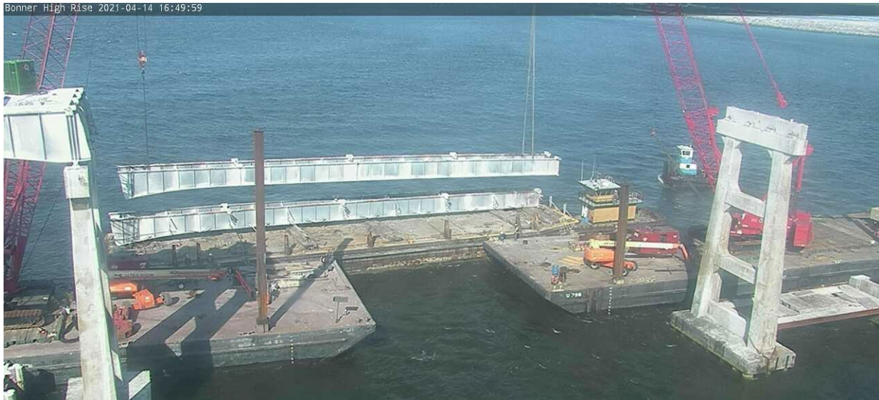
Figure 25 – Steel girders in Span 146 had been removed (photographed on 4/14/2021 by NCDOT)
