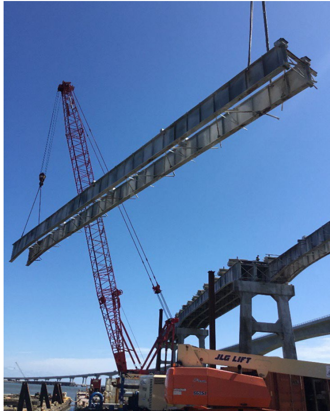
Figure 22 – Removal of Span 144 girders (photographed on 3/30/2021)
