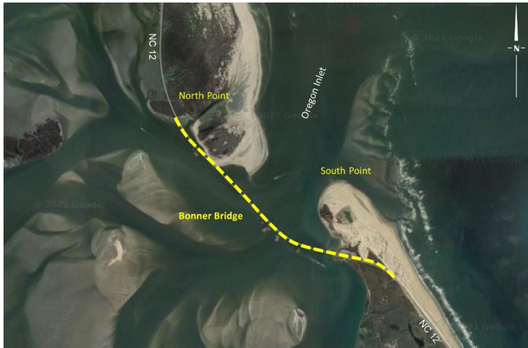
Figure 1 – Bonner Bridge (Modified from Google Maps)
