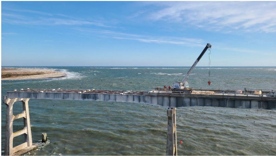
Figure 16 – Demolition of Spans 144 and 145 (photographed on 3/2/2021 by NCDOT)
