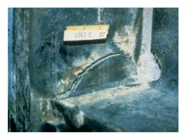
Damage ranges from small cracks that are difficult to see, to much larger cracks. Here, a crack began at the weld and progressed into the column flange, withdrawing a divot of material.
