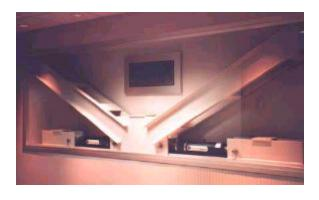
Energy dissipation systems are typically installed in buildings as part of a vertical bracing system that extends between the building's floors.
